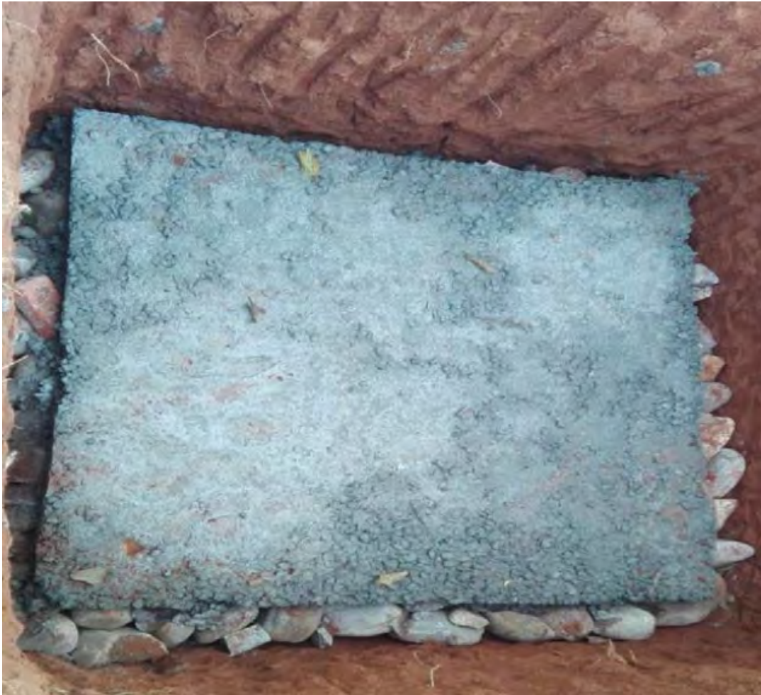
Photo 4: PCC on soling
