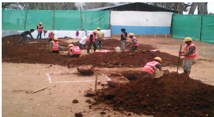
Photo 2: Earthwork Excavation
