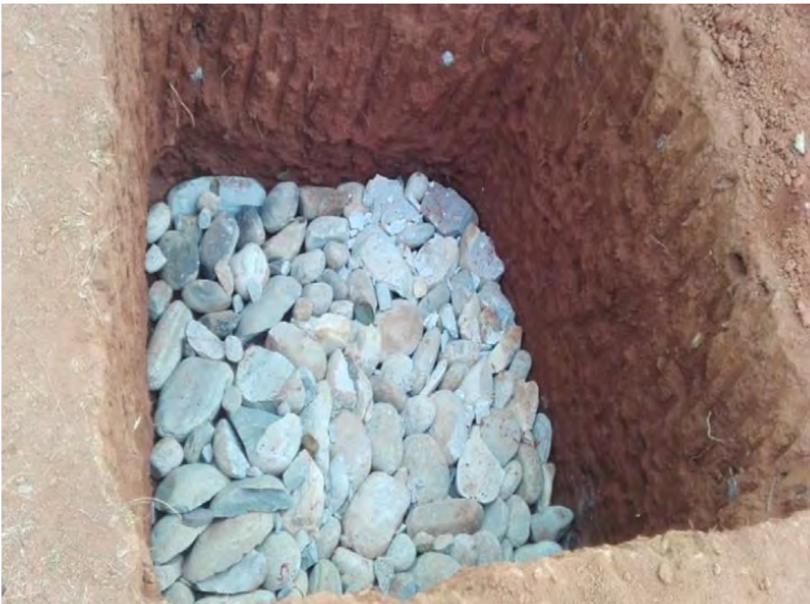
Photo 3: Boulder Soling on compacted earth
