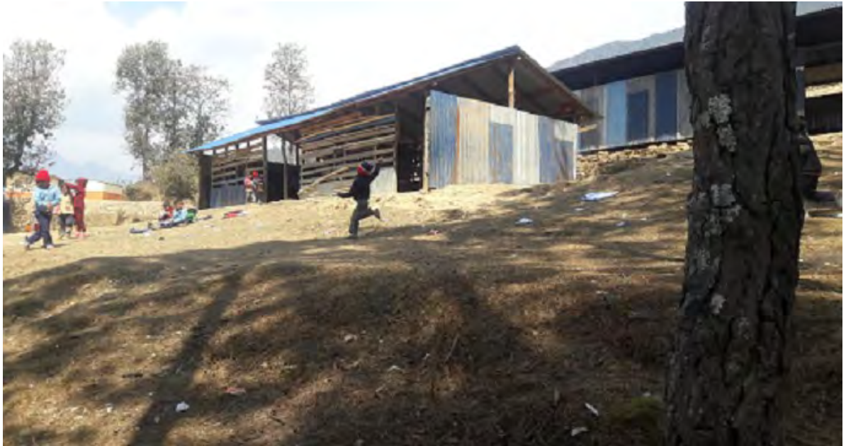
Photo 1: Existing site and TLC
