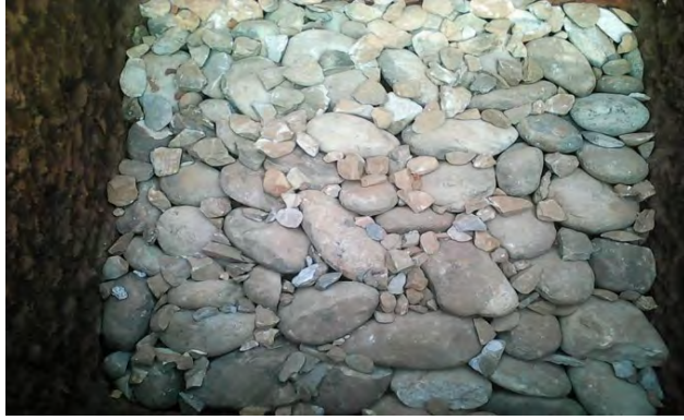
Photo 3: Boulder Soling on compacted earth
