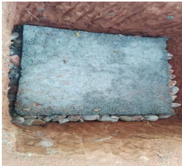
Photo 4: PCC on soling
