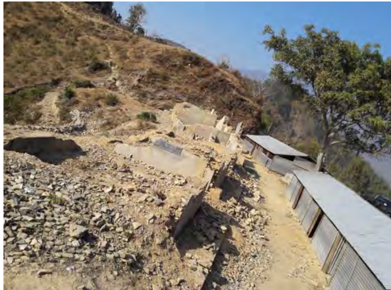
Photo: Dismantling of existing building
