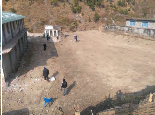
Layout works at site
