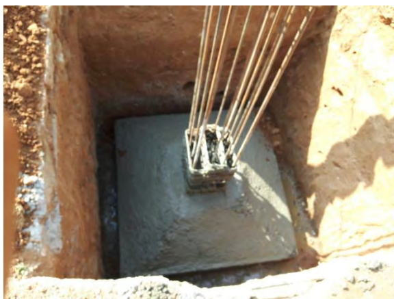
Column Bar with Footing
