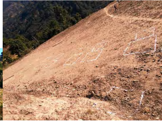
Layout works at site
