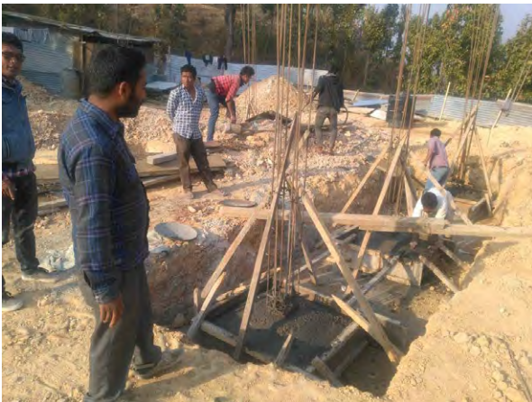
RCC works at footing of TC(S)
