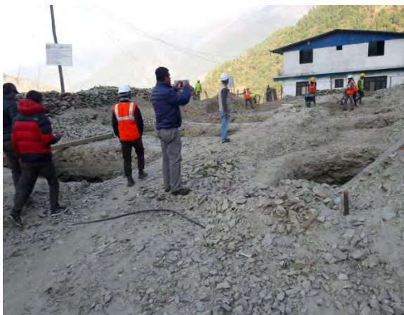
Foundation excavation with stone soling
