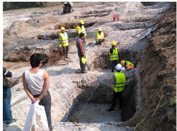
centering of column marks layout works
