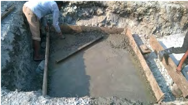
PCC works at site at 2-4C(S) and 2-4C(S)-A
