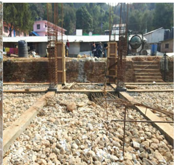
Tie Beam & column with flooring material
