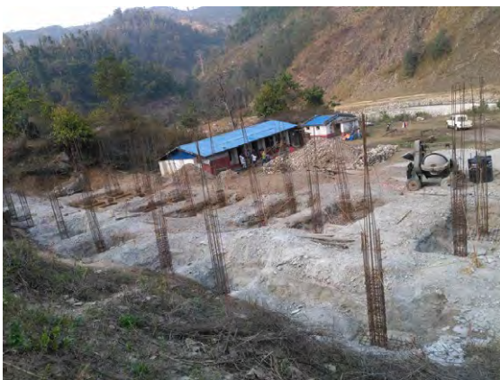
Erecting column re-bar at 2-4c(S) and 2-4C(S)-A
