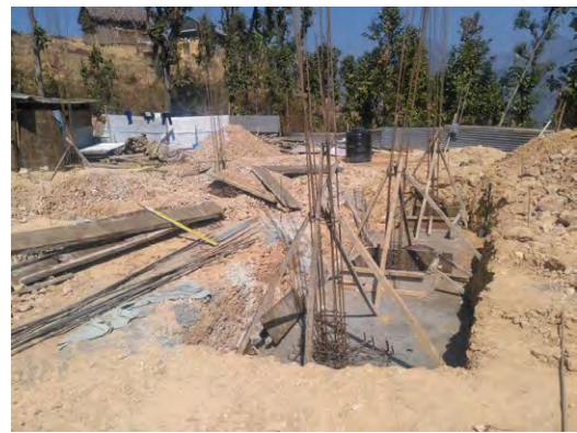
centering and leveling works
