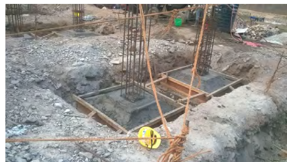
RCC work in footings of 2-4c(S) and 2-4C(S)-A
