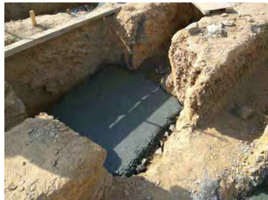
PCC works at TC(S)
