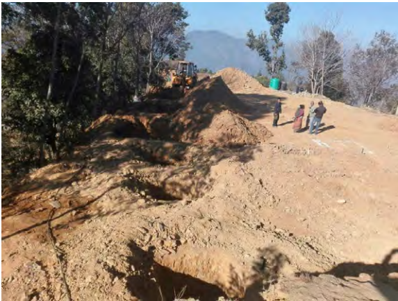
EW excavation work at 3-(C(S)
