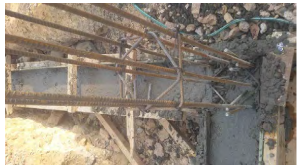
Lower tie beam rcc work at TC(S)
