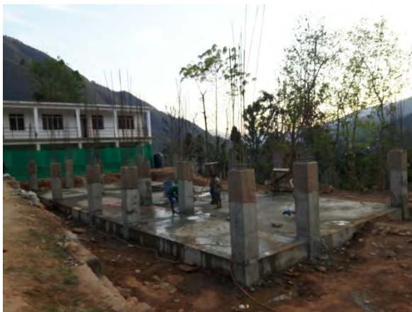
Plinth Level with column
