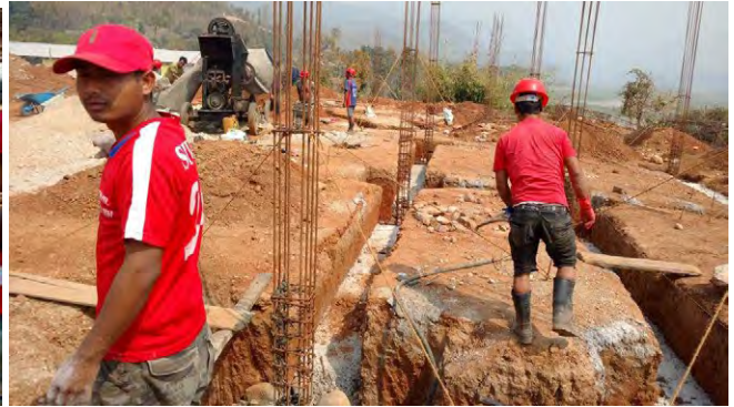
pcc works on trenches of TC(S)
