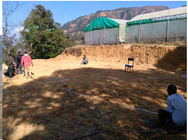
Foundation layout works
