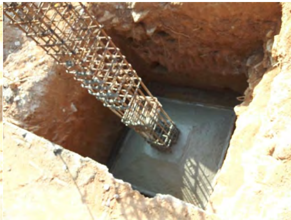
Column Bar with Footing
