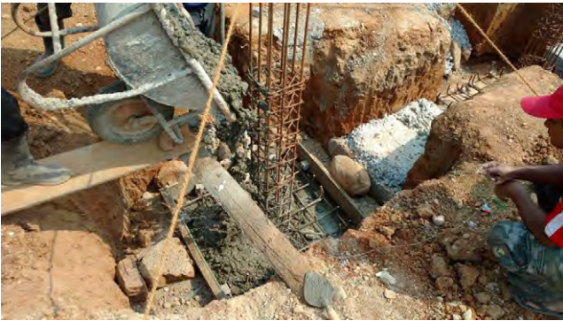
RCC works at footing of TC(S)
