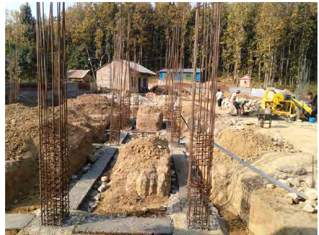
Trench soling and pcc works at 2-4c(S)
