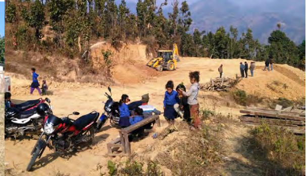
site preparation works
