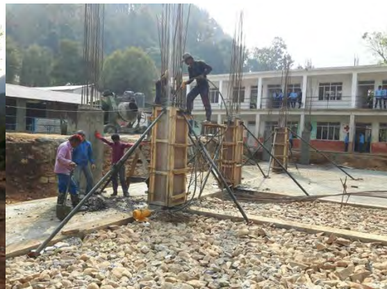
Form work of Column
