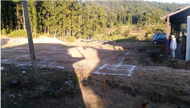
Layout works at site
