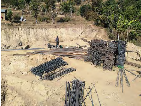
Re-bar works at site
