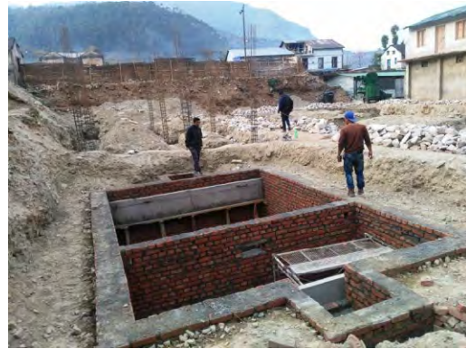
septic tank construction
