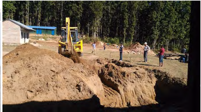
EW excavation works
