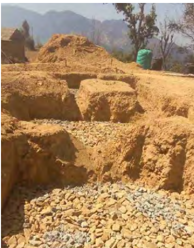
Stone soling work at 3-9C(S)
