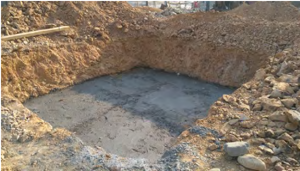
Pcc works at 2-4c(S)
