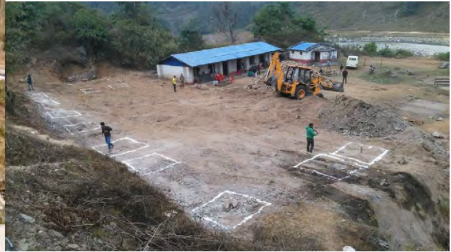
Foundation layout works
