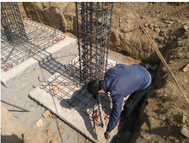
Leveling and centering works at 2-6c(S)
