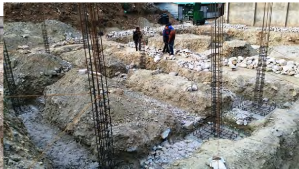
Re-bar works at tc(M)
