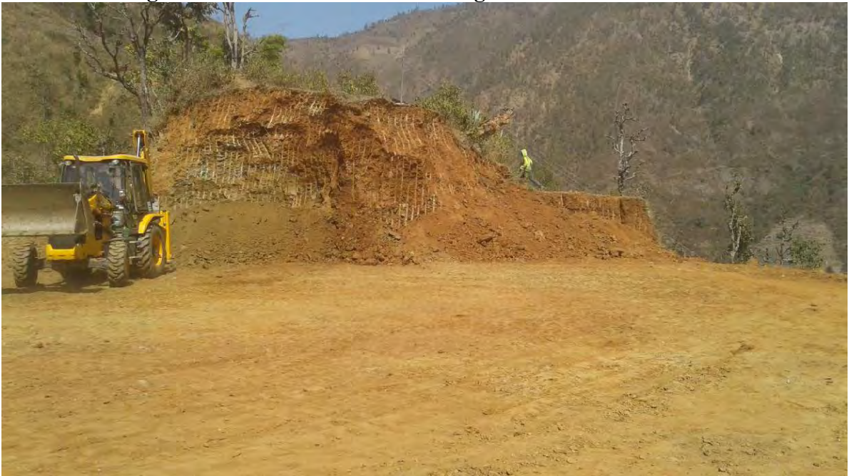
Picture showing 3 m level after earthwork cutting:
