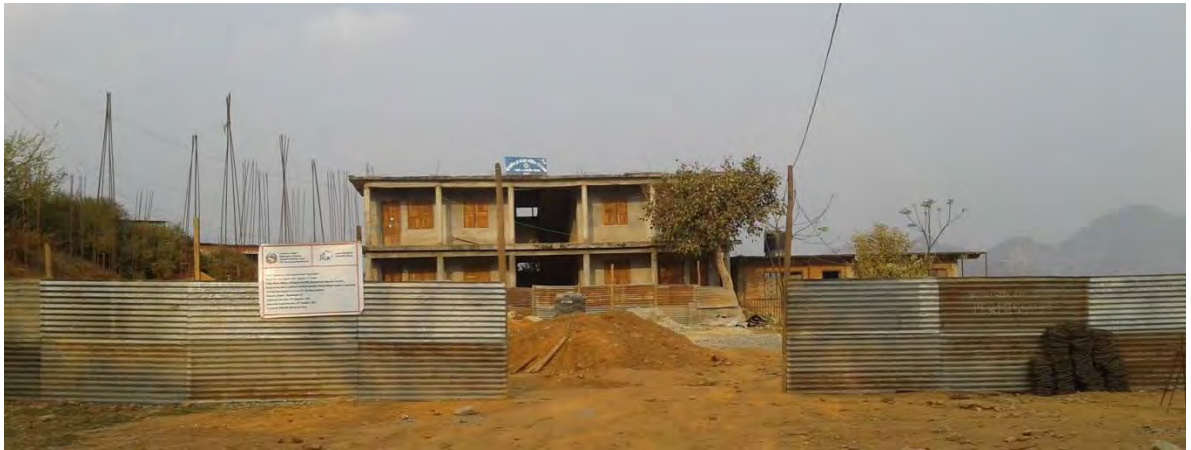
Figure 2 : Shree Shanti HS School Site
