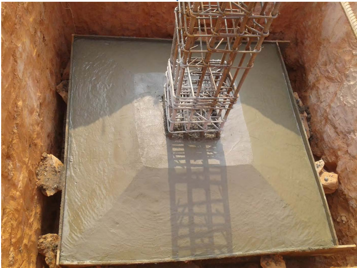
Figure 4 : Column footing cast of Practical Block, 2-LaLi 2CM
