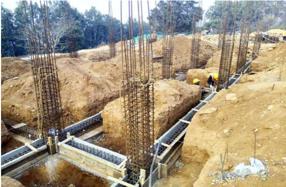
Figure 4 : Rebar and formwork of LTB of Academic Block 1
