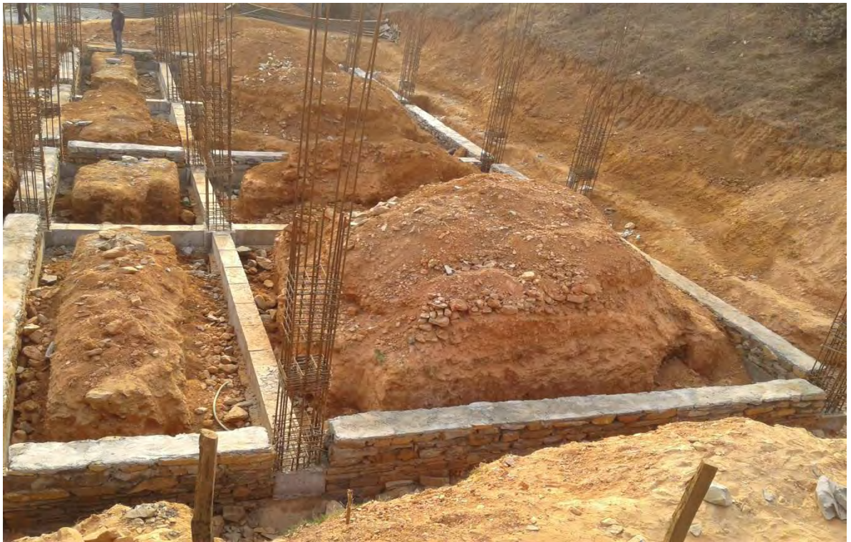
Figure 3 : Stone Masonry works above LTB of Academic Block, 2-6C (S)
