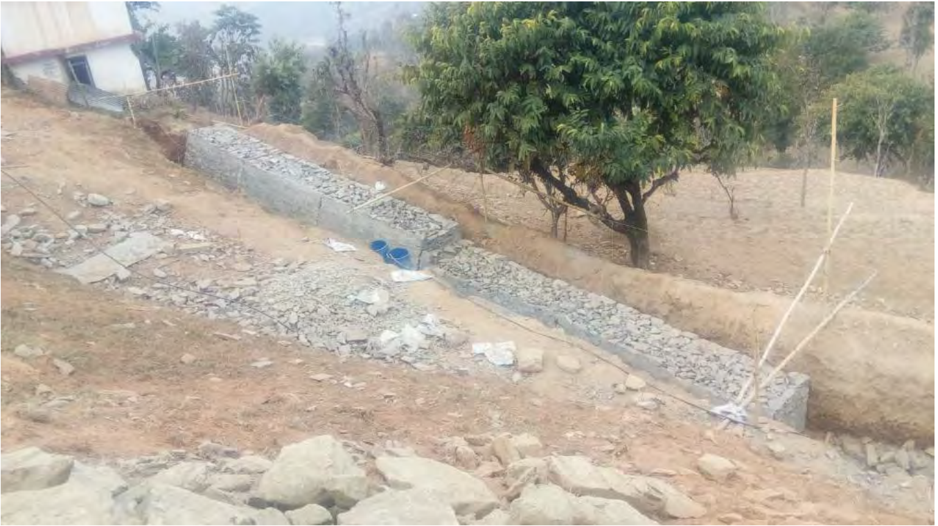
Figure 4 : Site Development Works i.e. Retaining wall
