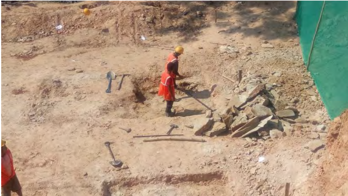
Figure 7 : Footing excavation of Multipurpose Block M (S)
