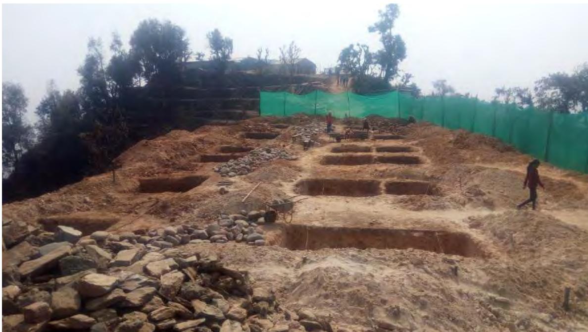
Figure 6 : Footing Excavation of Practical Block, 2-LaLi 2CM
