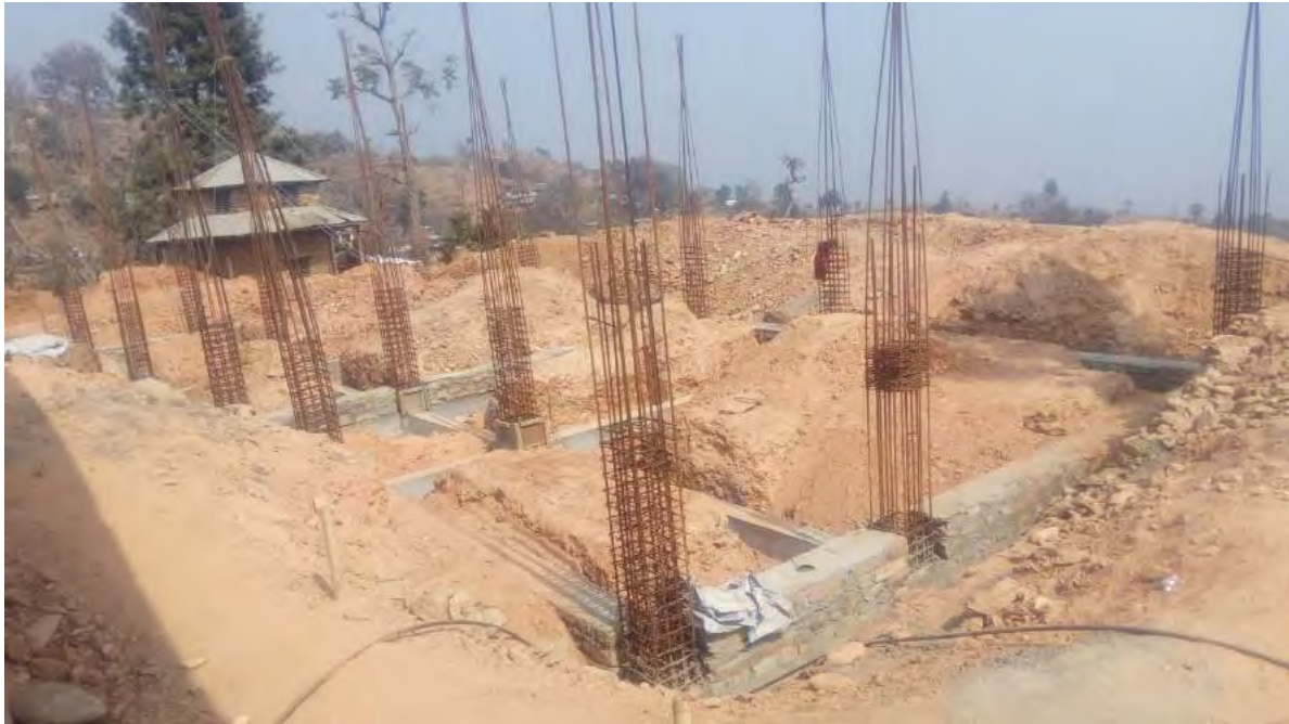
Figure 5 : Stone Masonry wall below UTB of 2 nd Academic Block, 2-6C (S)
