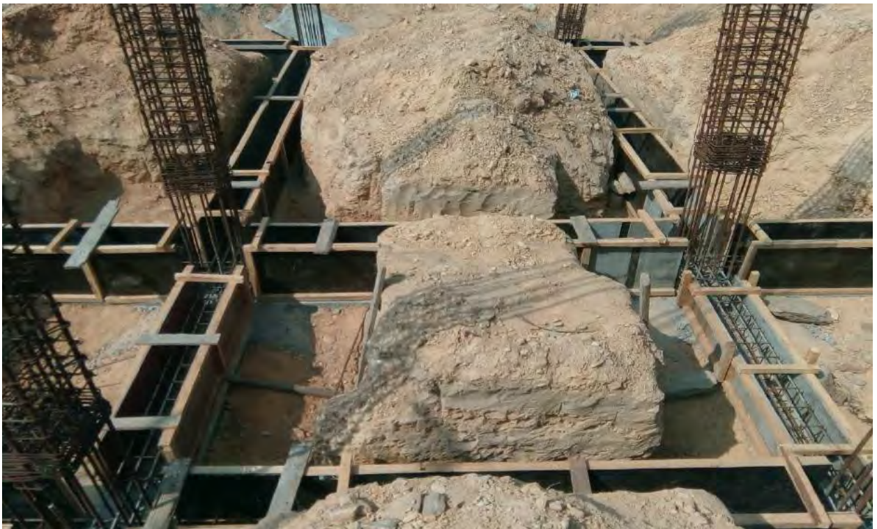
Figure 3 : Rebar & formwork of LTB in Academic Block, 2-4C(S)
