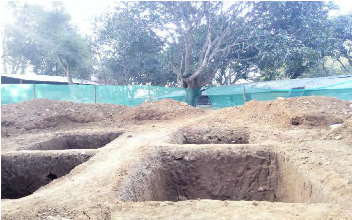
Figure 6 : Earthwork excavation of Practical Block
