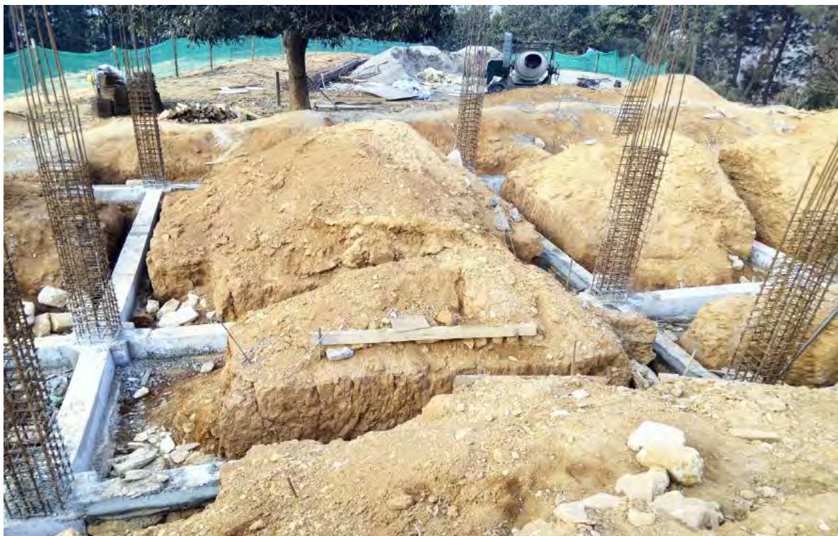
Figure 5: Stone masonry works below LTB of Academic Block-2
