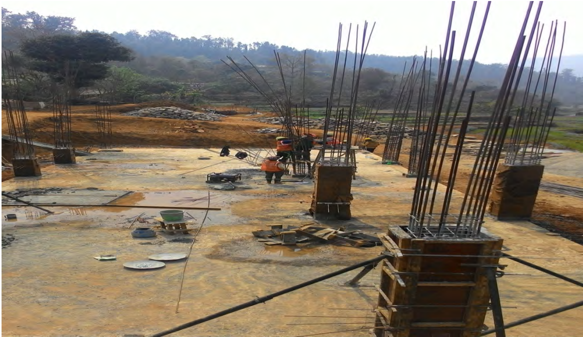
Fig: Ground floor Column Work
