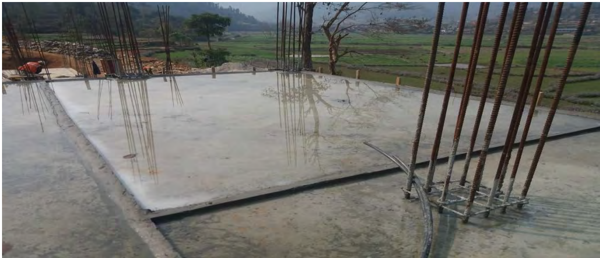
Fig: Curing of first floor slab level
