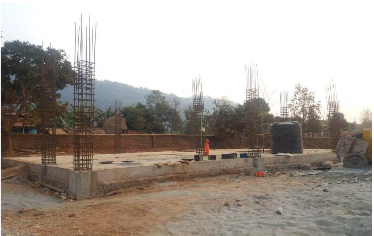
Fig: Reinforcement work Ground floor column
