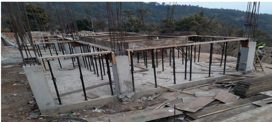
Fig: Form work for first floor level
