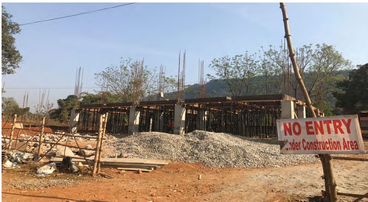
Fig: Form work for first floor level
