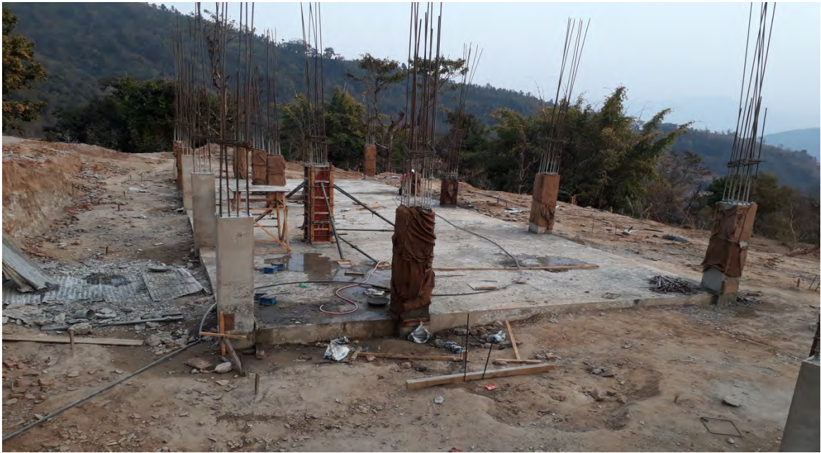
Fig: Curing of ground floor column
