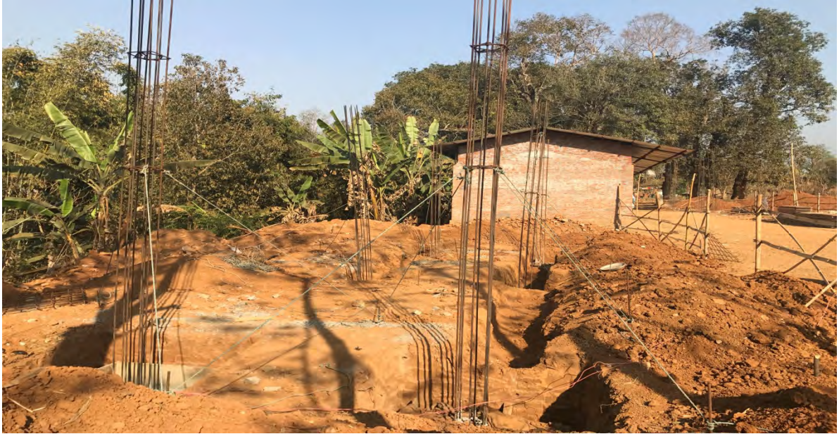
Fig: Excavation work for lower tie beam
