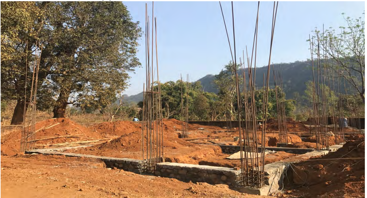
Fig: Stone masonry work between lower and upper tie beam
