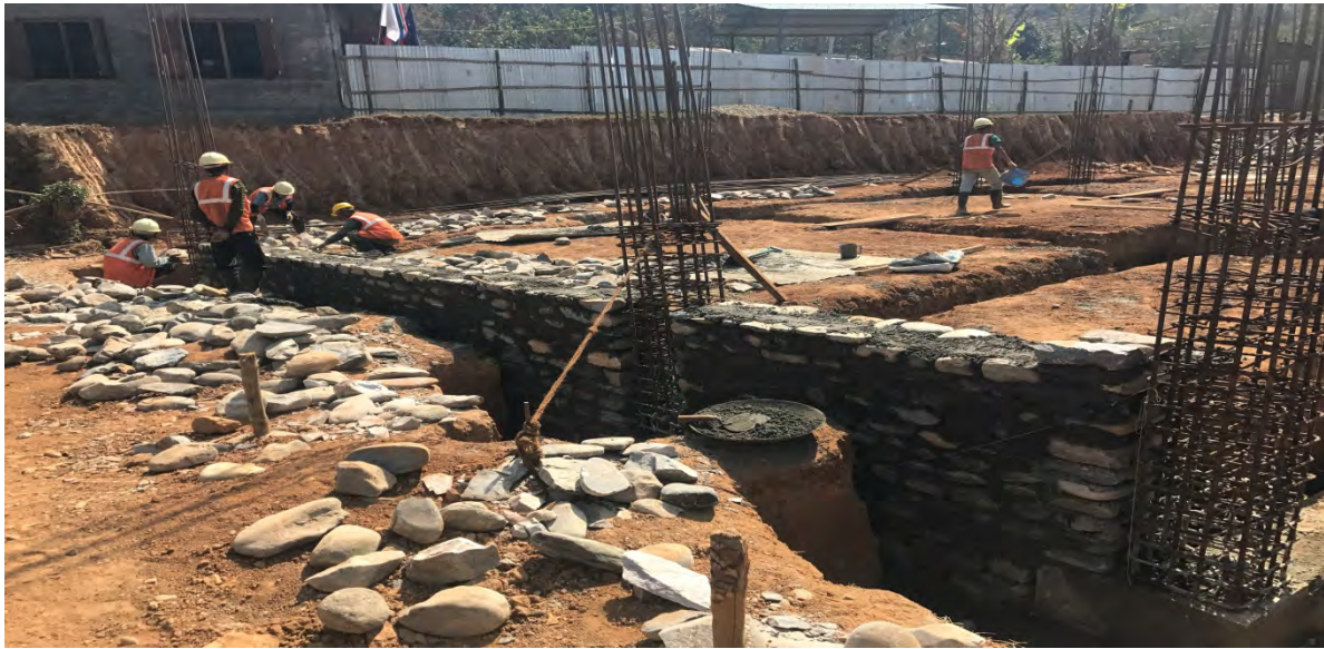
Fig: Stone masonry work between lower and upper tie beam
