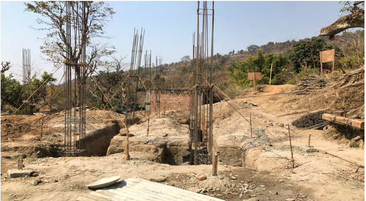
Fig: Excavation work for lower tie beam
