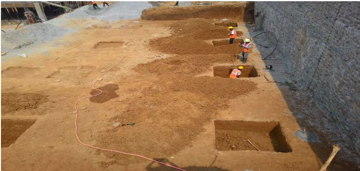
Fig: Excavation work for foundation
