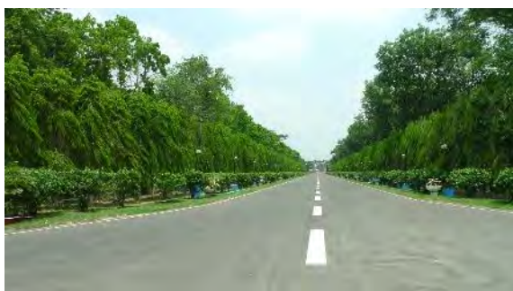
VVIP Terminal Entrance Access Road Source: JICA Study Team
