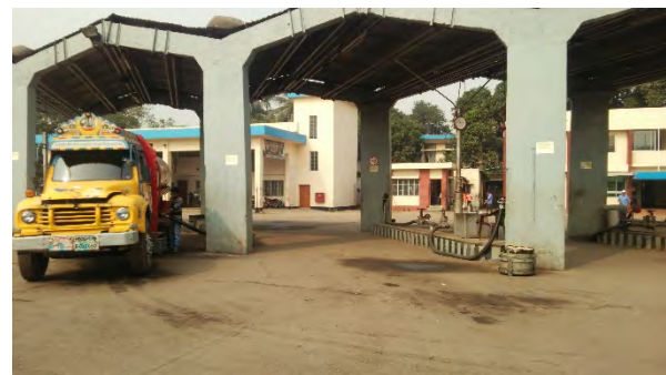
Existing Tank Truck Receiving Facilities
