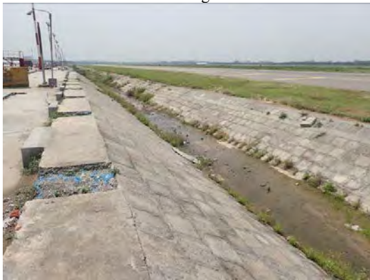
Existing Open Channel
