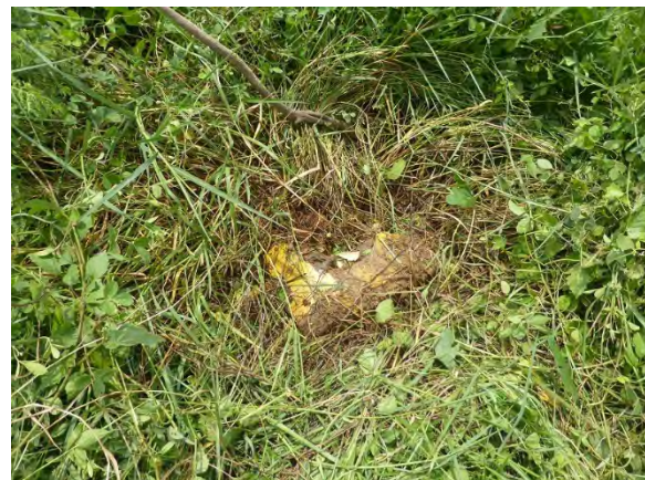
Temporary Benchmark (Damaged)
