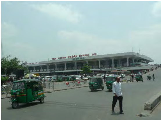
Existing Terminal 1 and Terminal 2 Exterior Source: JICA Study Team
