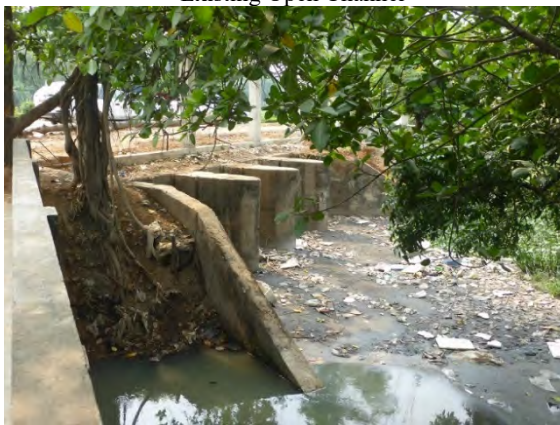
Drainage at the Southeastern Corner
