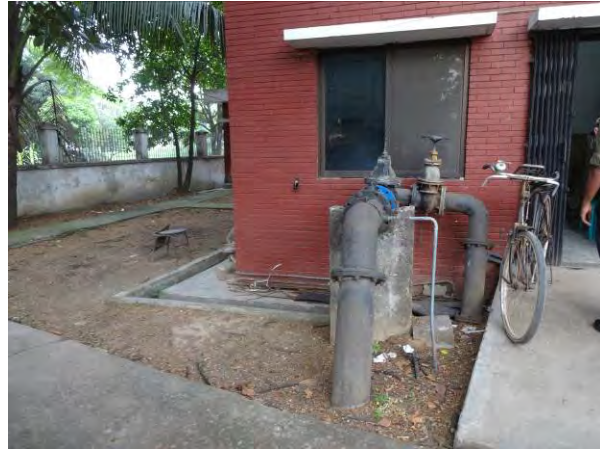
Figure 3-36 Existing Water Supply
