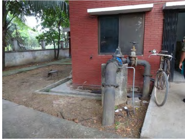
Figure 3-36 Existing Water Supply
