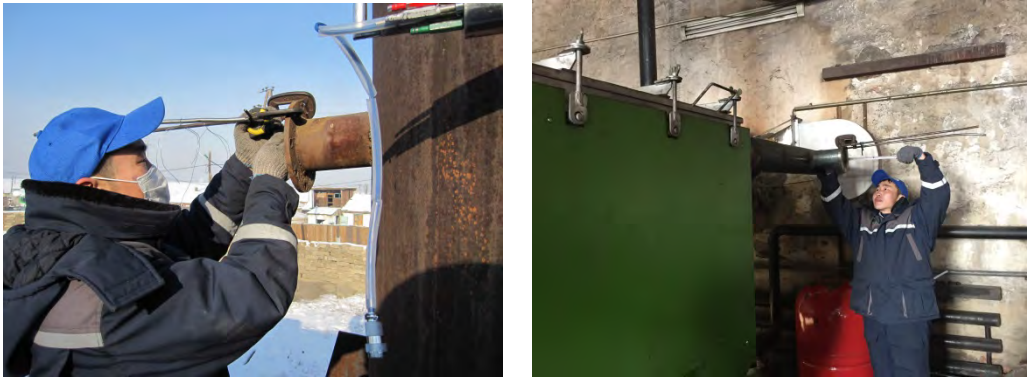
Figure 8-20 Measurement of Size of Measurement Hole
