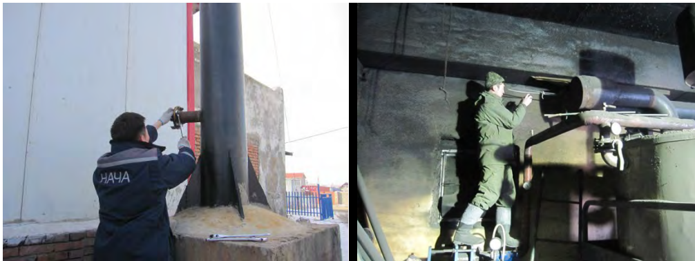
Figure 8-19 Opening of the Measurement Hole and Cleaning
