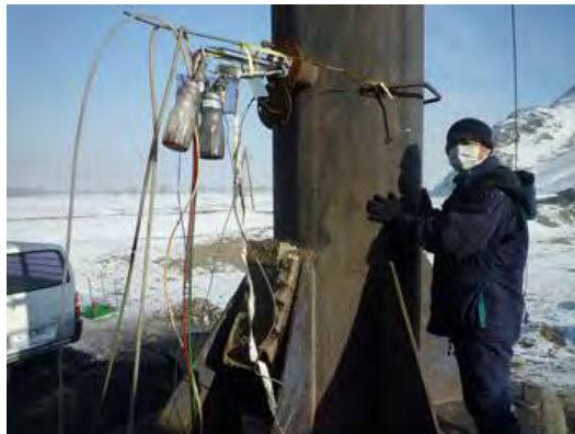
Figure 10-4 Installed Equipment on the Chimney Side (For the Automated Equipment)
