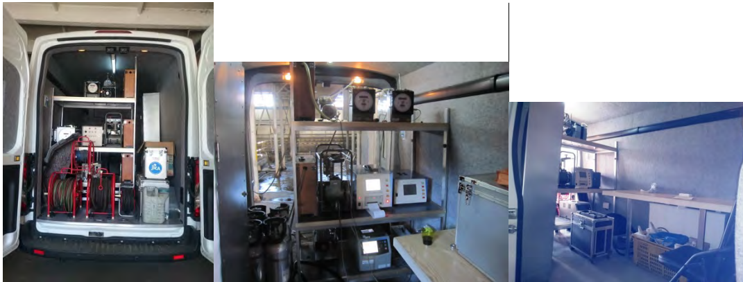
Figure 8-1 Loading of the Instruments
