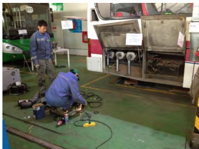
April 2015: Installation of DPF (bus)
