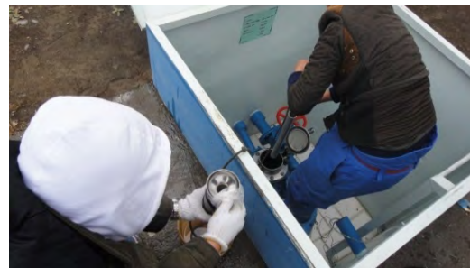
October 2014: Obtain fuel from warehouse
