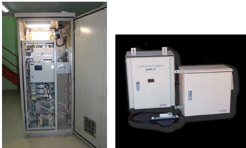
Figure 2.5-2 Flue Gas Measurement Analyzers and Dust Analyzer
