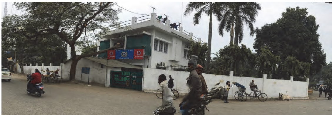
Figure 5.3.11 South East Corner – CRPF Mess Building
