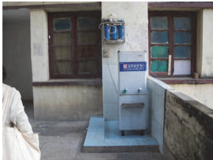
Figure 5.3.28 Potable water equipment with filter
