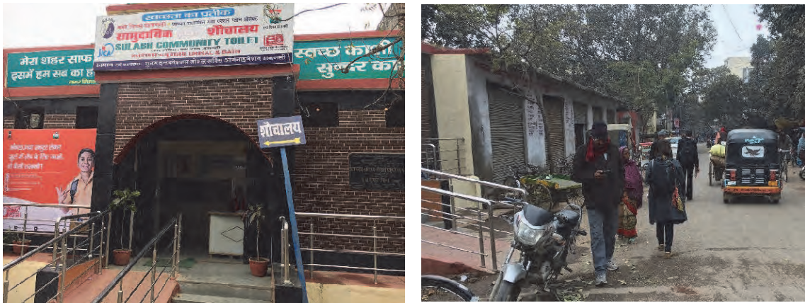
Figure 5.3.18 West Side –JICA Funded Public Bath & Toilet (left) and West Side – Community Stores (right)
