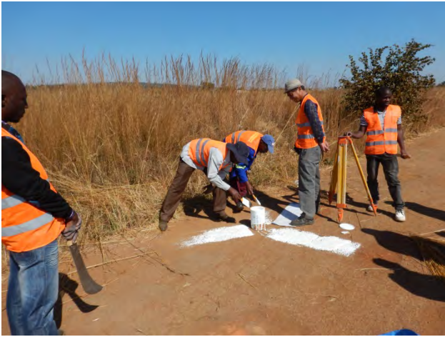
Training on an air mark installation
