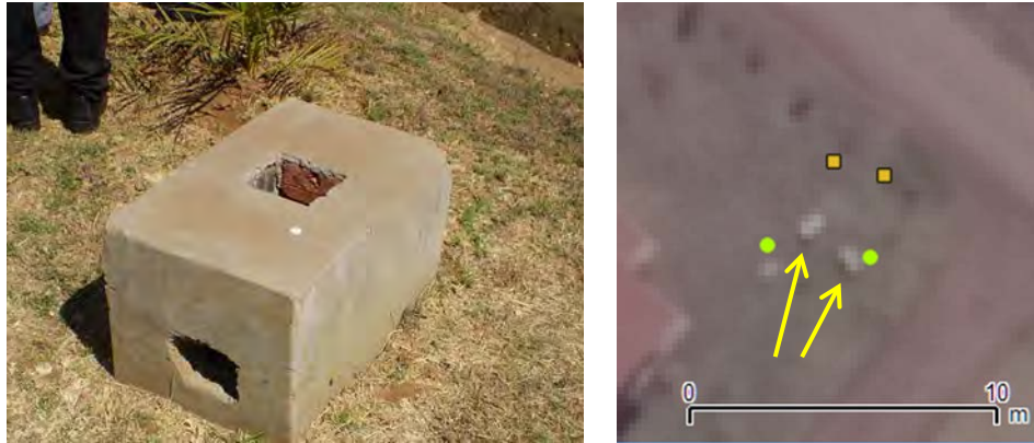
Figure 42 Appearance of water meter concrete box (left) and yellow arrows indicating water meter box on digital orthophoto (right)
