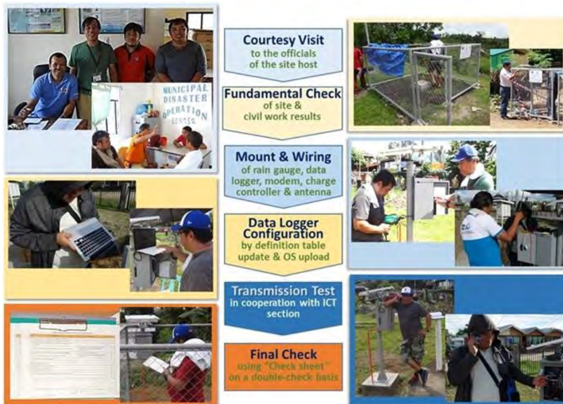
Fig. 3-3-12 Procedures of on-site work for ARG installation
