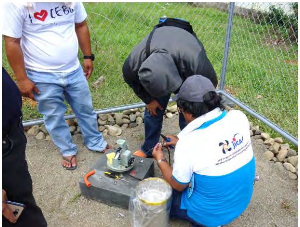
ARG Installation Work (Output 2a)
