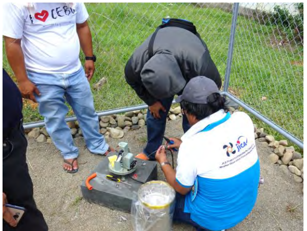
ARG Installation Work (Output 2a)
