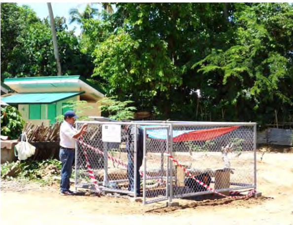
ARG Installation Work (Output 2a)
