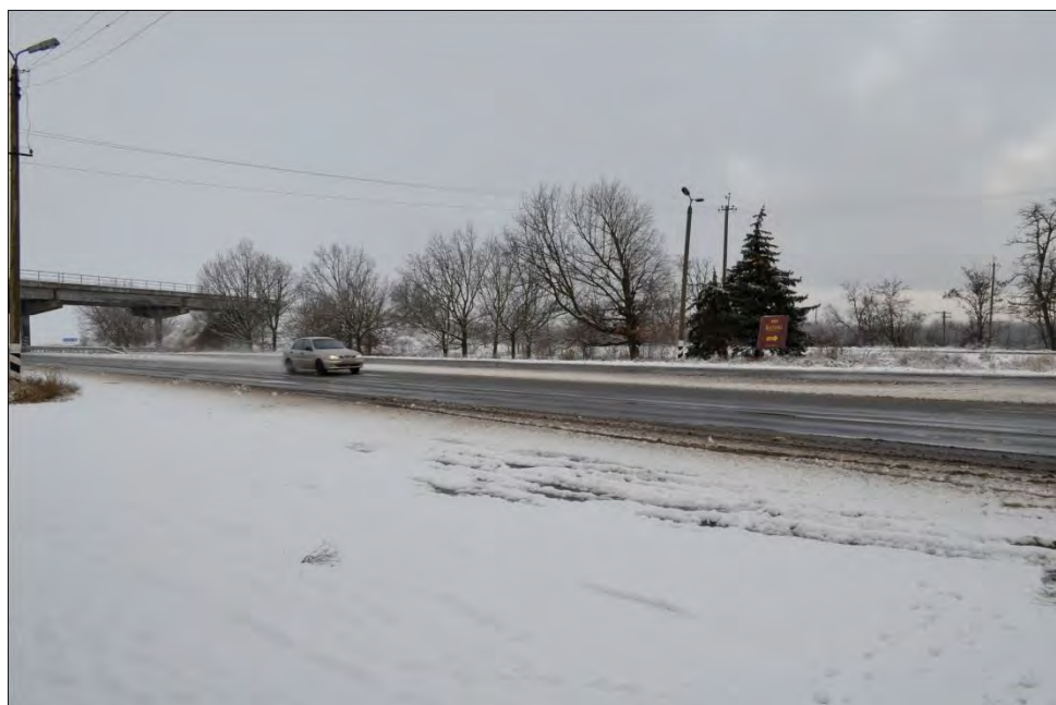
Figure 25 The camera coverage at Traffic Volume Survey Location 2 (road M14 towards Polovynky settlement)
