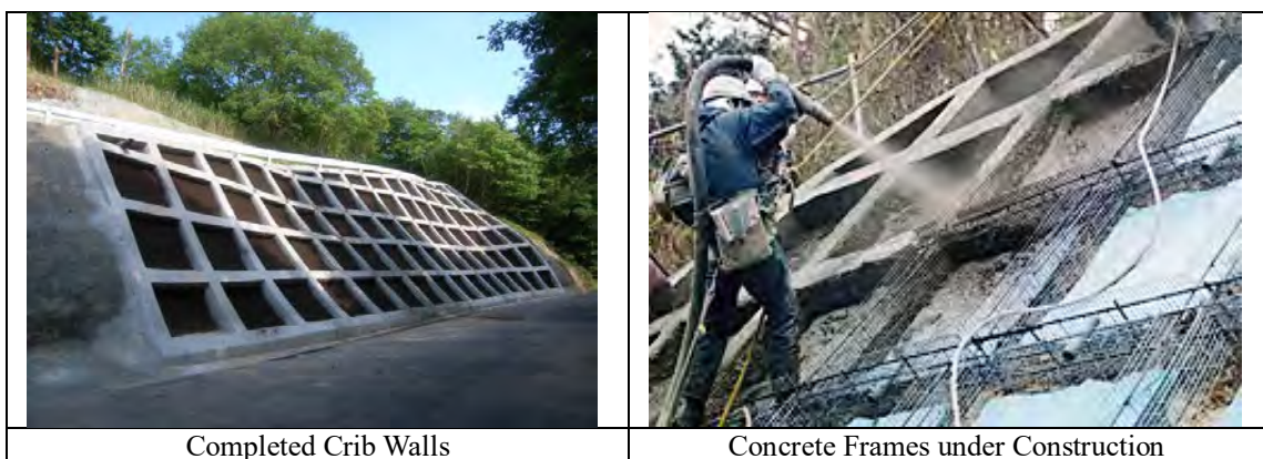
Figure 8.7 Slope Protections Using Concrete Frames
