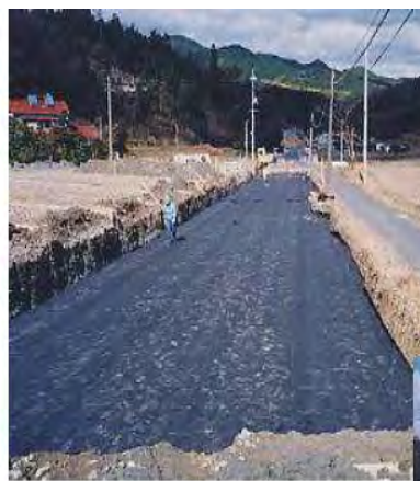
Figure 8.2 Photo of Laying of Geo-Textile on the Ground
