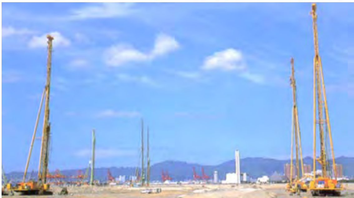
Figure 8.59 Sketch and Picture of Sand Drain
