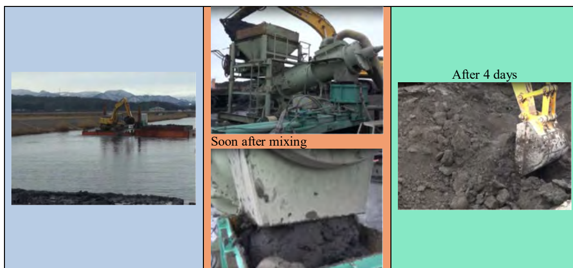
Figure 8.58 Detailed Construction Procedure of Cement Mixing Method
