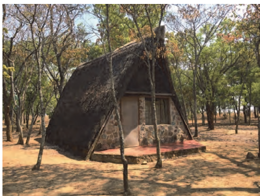
Accommodation building (Chalet)
