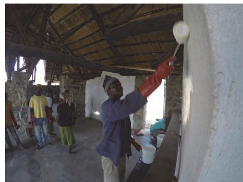
Re-painting of walls
