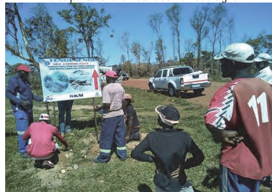
Installation of a road sign
