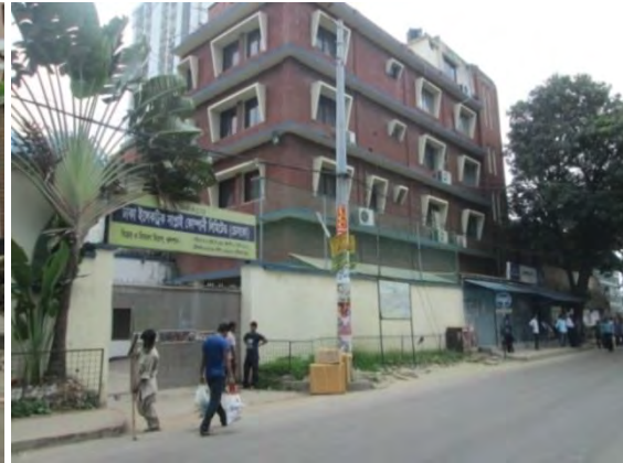
Northern side of the project location
