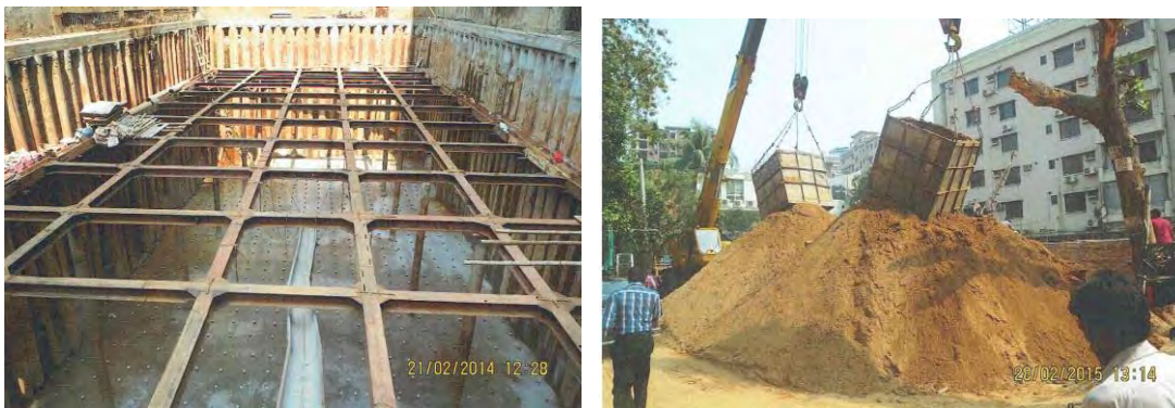
Figure 2-25: Example Pictures of Construction Stage of Underground Structure (Earth Support System and disposal of Excavated Material)
