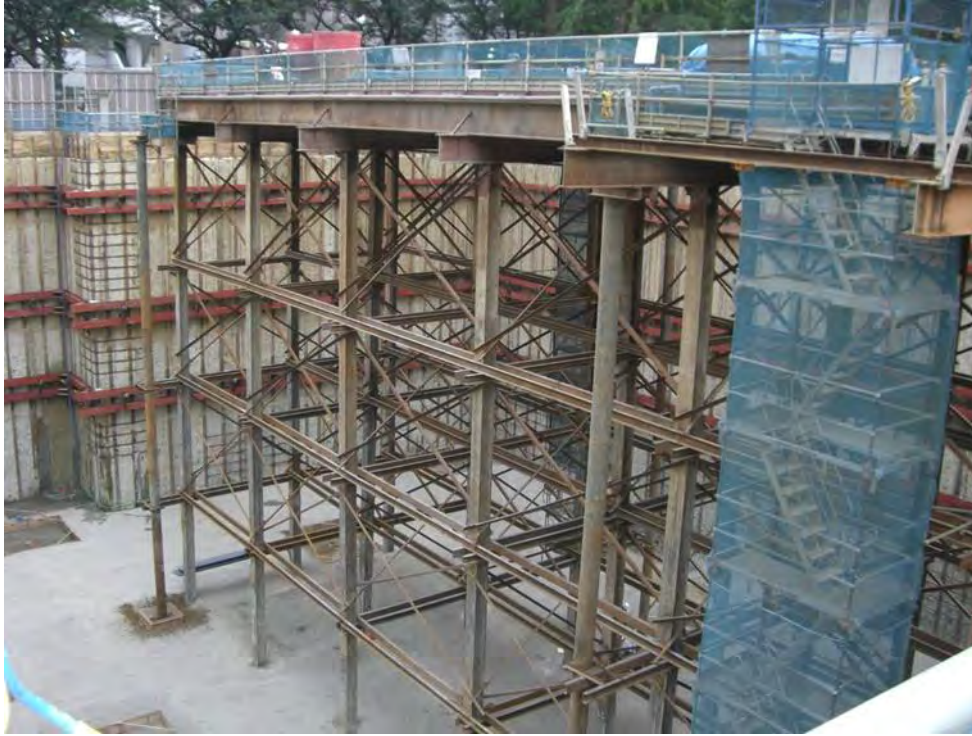
Figure 4-19 Example of Temporary Staging
