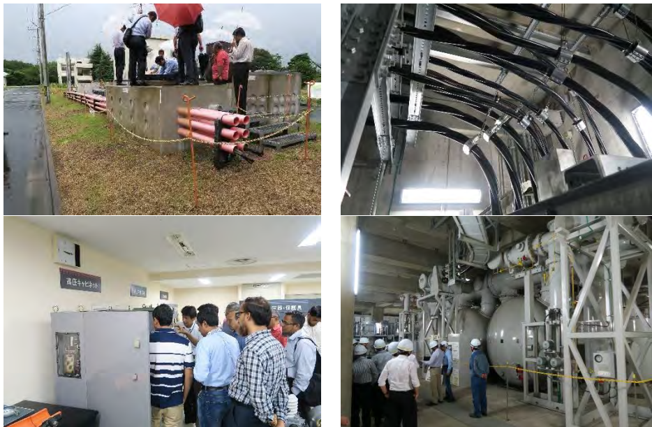
Figure 1-5 Pictures of On-site Visits
