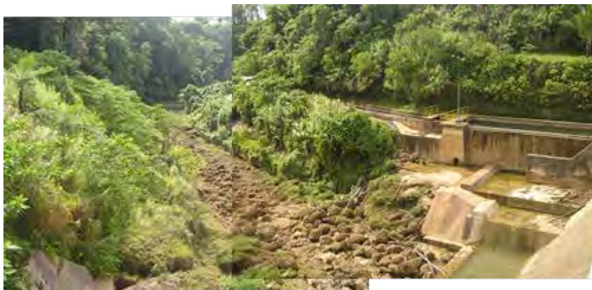
Picture 5-2-7 River Condition, Downstream of the Weir (Overspill=0)
