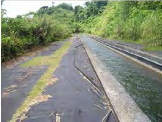
Picture 5-2-10 Water Channel, Surface Drainage Sheet
