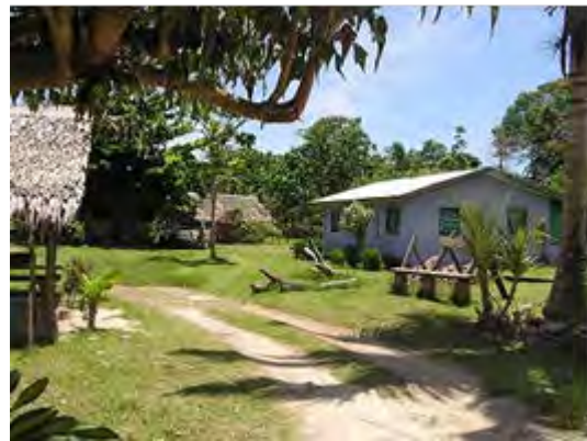
Picture 5-6-6 Undistributed Settlement, Located Several Kilometers from the Left Low-Volatage Distribution Point
