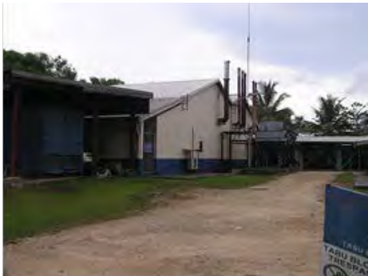
Picture 5-3-1 Diesel Generator Power House
