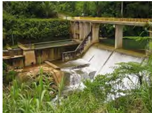
Picture 5-2-2 Intake Weir with Settling Basin, Downstream Side
