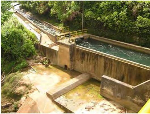
Picture 5-2-5 Settling Basin and Water Channel
