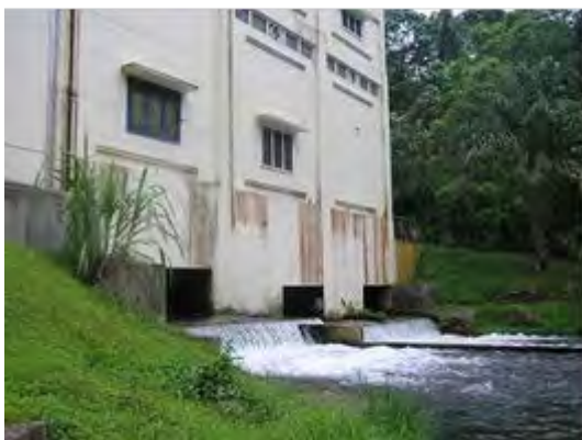
Picture 5-2-20 Powerhouse Tailrace
