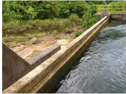
Picture 5-2-6 Settling Basin Spillway Section Bulk-up Condition
