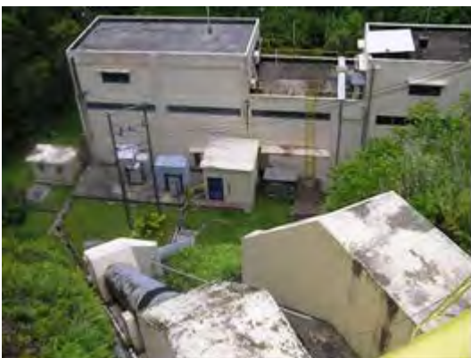
Picture 5-2-14 Penstock (View from Headtank)
