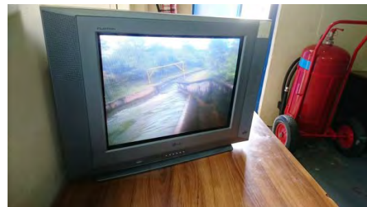
Picture 5-2-19 Spillway Monitor
