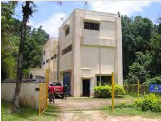
Picture 5-2-16 Power Houser Building
