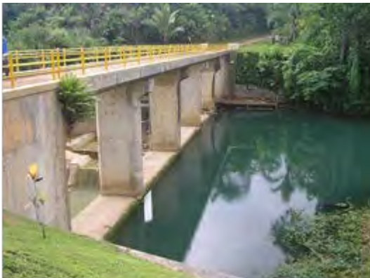
Picture 5-2-1 Intake Weir, Upstream Side
