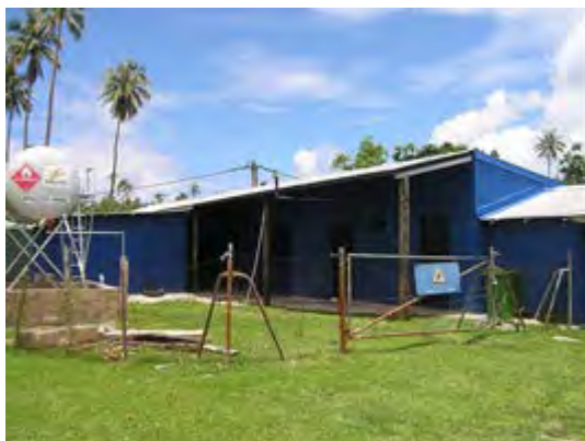
Picture 5-4-1 Overview of Power Plant
