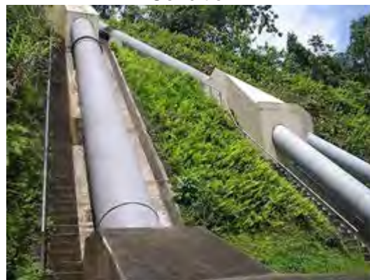
Picture 5-2-15 Penstock (View from Power House)
