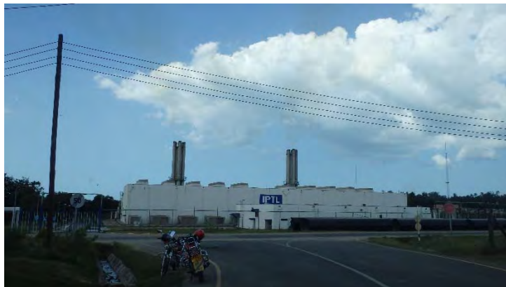
Figure S-1-1.4 Tegeta IPTL Thermal Station (IPP Unit)
