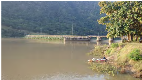
<Reservoir and Front Face of Dam>
