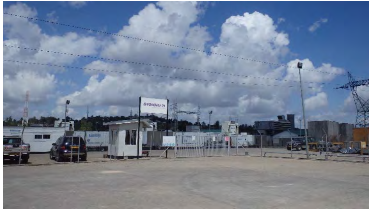
Figure S-1-1.5 Symbion Ubungo Thermal Plant (EPP Rental Unit)
