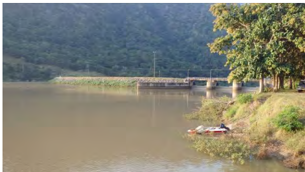
<Reservoir and Front Face of Dam>
