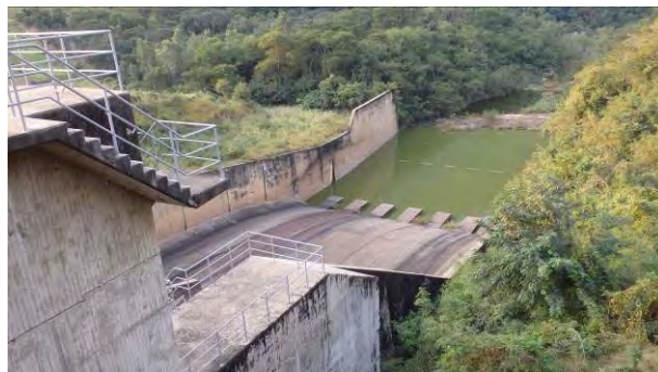
<Spillway of Dam>
