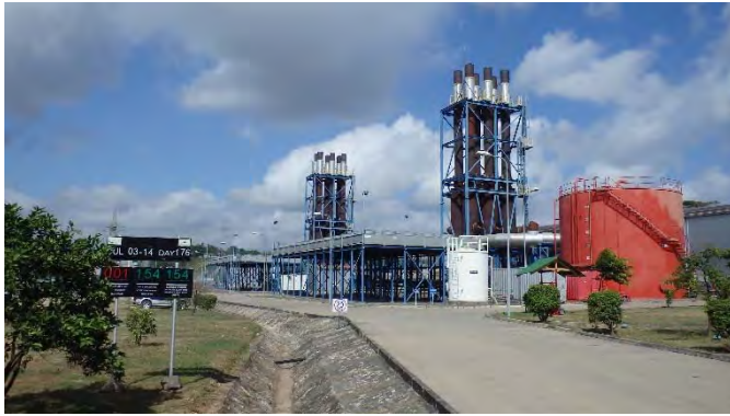
<Overview of the plant>
