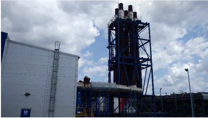
<Overview of the plant>
