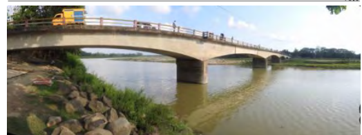
Matamhuri River Bridge (along NR-1)
