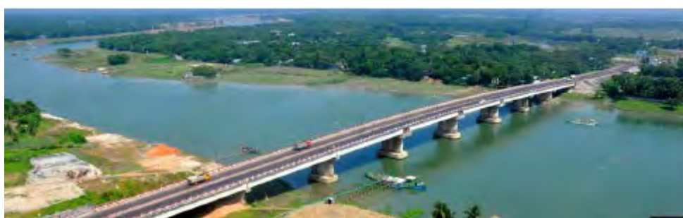
Figure 4.4.3.3 Kanchan Bridge (Shitalakshya river crossing bridge, right side of figure towards to Araihasar EZ)
