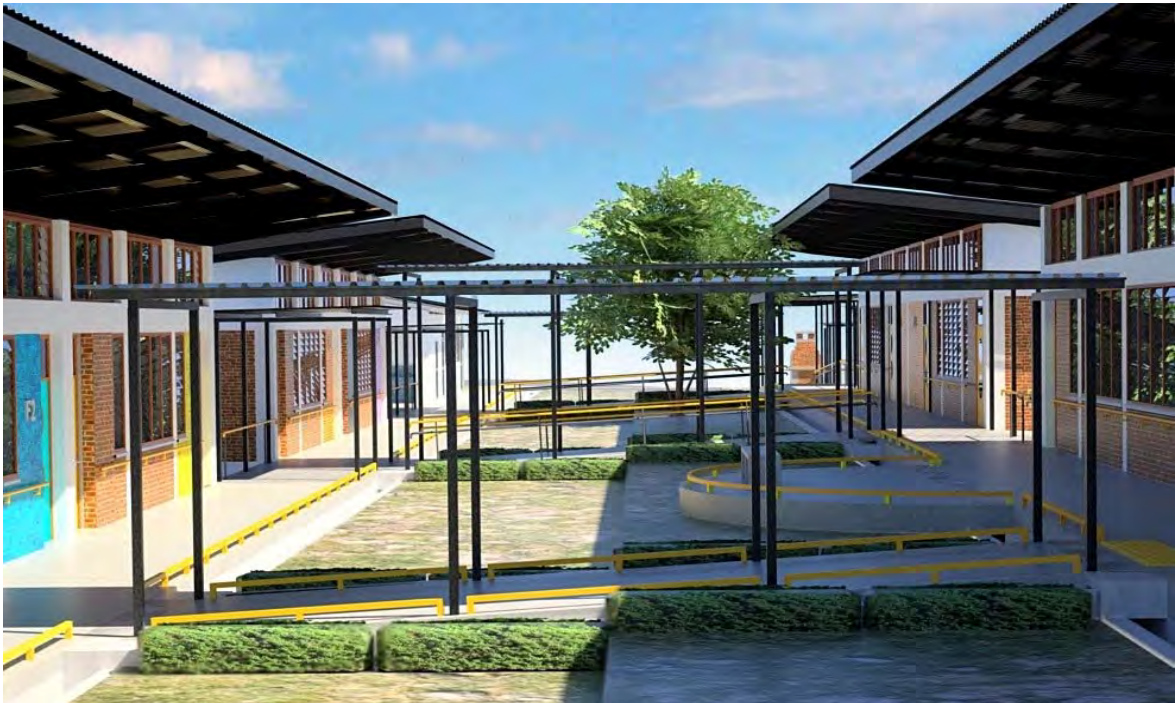
Aspect of Project Facilities (S1 Eqiniseni)
