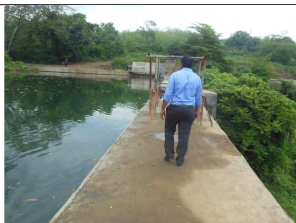
Water intake dam
