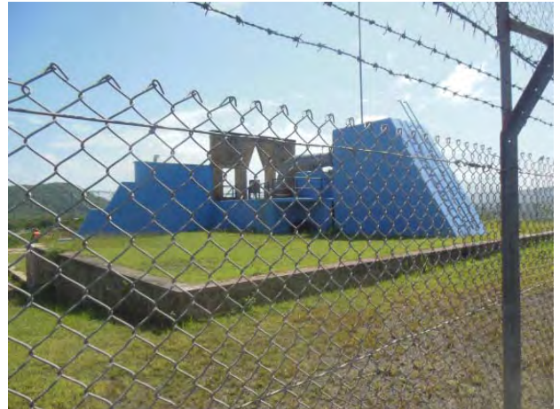
Gravity pipe from station to city
