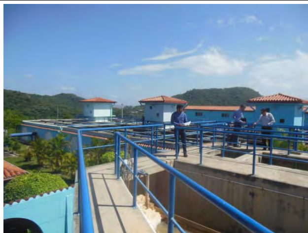
Overview of plant from inlet side
