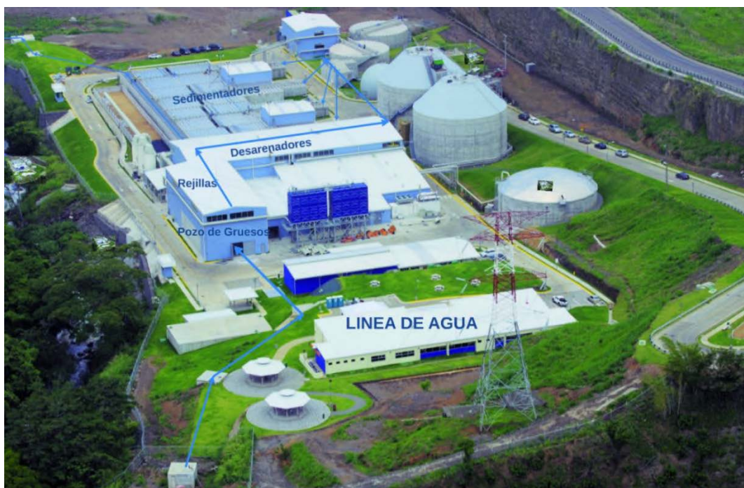
PTAR “Los Tajos”
