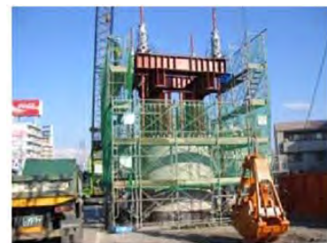
Construction of Caisson Structure
