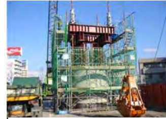
Construction of Caisson Structure
