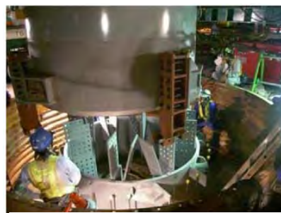
Connection part at tip of pier column
