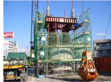
Construction of Caisson Structure
