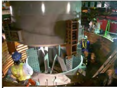
Connection part at tip of pier column
