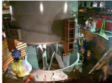
Connection part at tip of pier column
