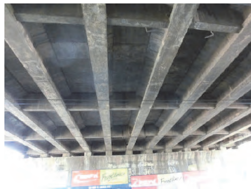
Photo 3.7.31 General View of Goregaon ROB
