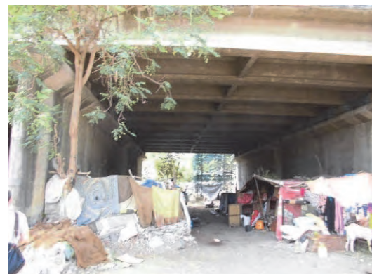
Photo 3.7.34 Squatters under the ROB in Western Railway site
