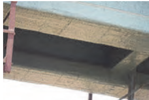
Photo 3.7.68 CFRP Epoxy Coating
