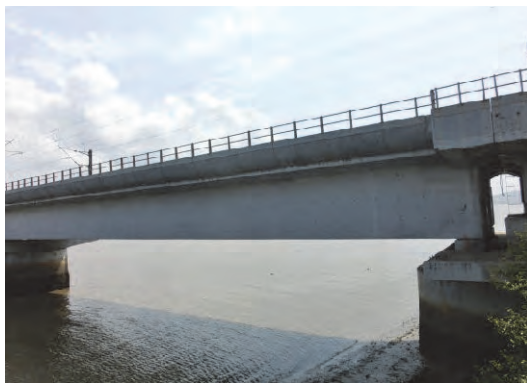
Photo 3.7.49 General View of No. 73 Bridge
