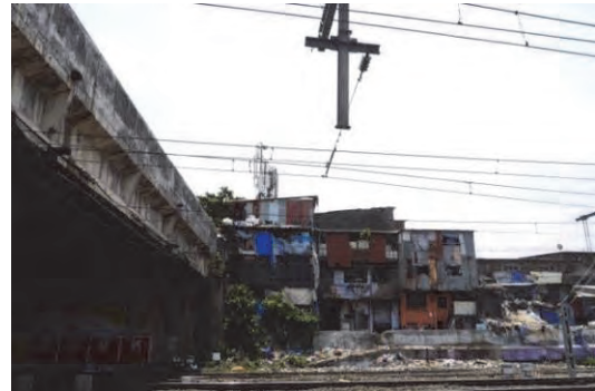
Photo 3.7.28 View of Southeast side from ROB
