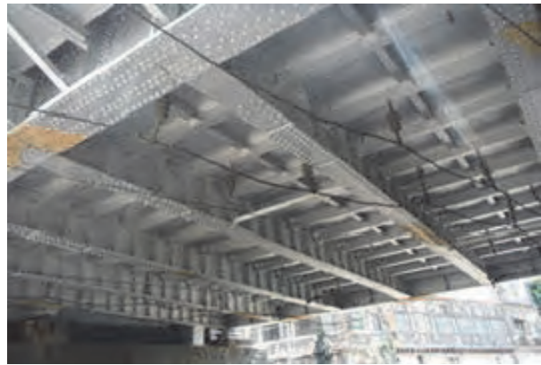
Photo 3.7.2 Main Girder and Cross Beam
