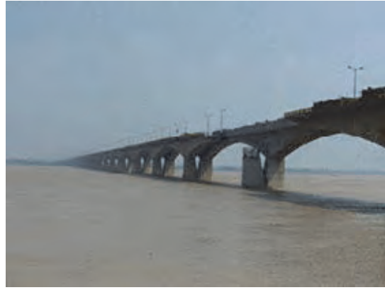
Photo 3.6.2 Removal of existing Superstructure from existing Mahatma Gandhi Bridge
