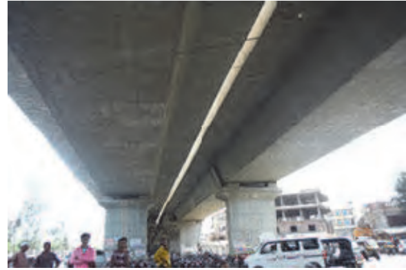
Photo 3.7.36 General View of LC No.5/A
