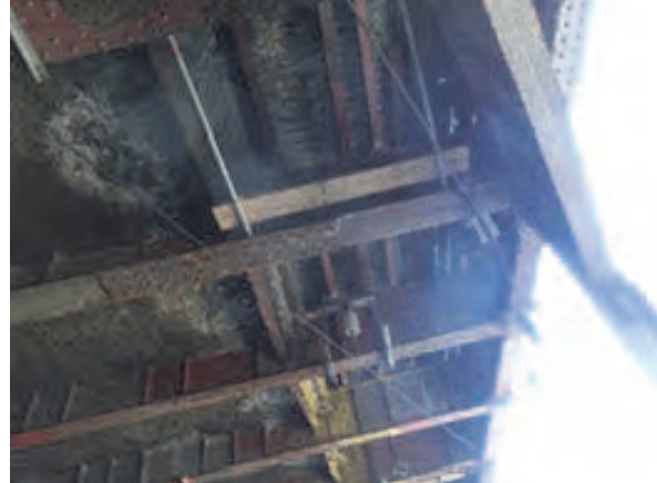
Photo 3.7.16 Peeling and Free Lime of concrete from Bottom of Deck Slab
