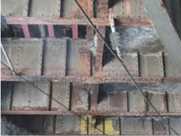
Photo 3.7.15 Rusted and Lack of Section at Bottom Flange
