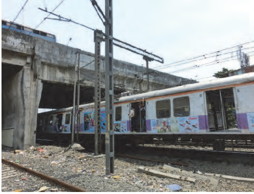
Photo 3.7.23 General View of Mahim Bridge
