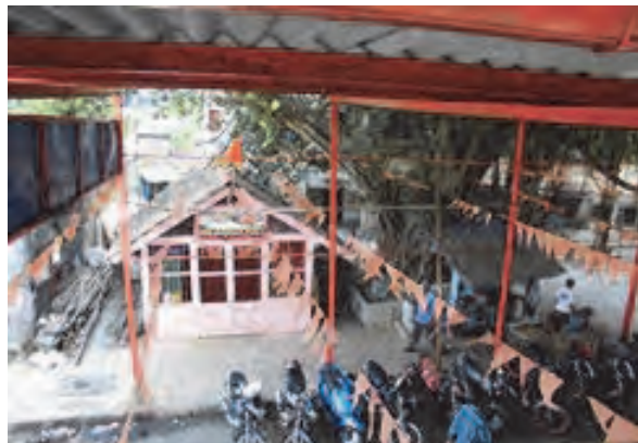
Photo 3.7.18 Temple on Southeast side from ROB
