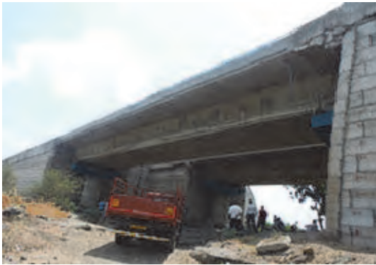
Photo 3.7.43 General View of LC No.2/A North
