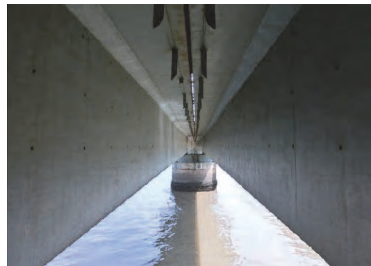
Photo 3.7.50 Between each Girder
