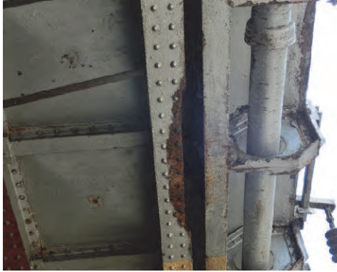
Photo 3.7.8 Lack of Section at Bottom Fringe
