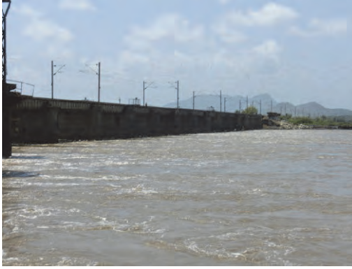
Photo 3.7.56 General View of No. 92 Bridge
