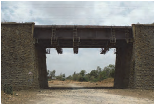
Photo 3.7.80 General View of No. R8 Bridge
