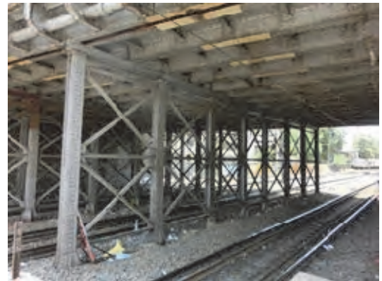
Photo 3.7.7 Girder and Pier Column
