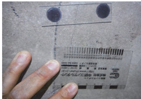
Photo 3.7.38 Cracks of Deck Slab
