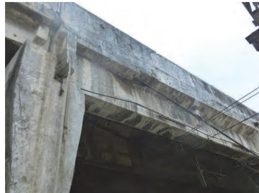
Photo 3.7.25 External Prestressed Cable
