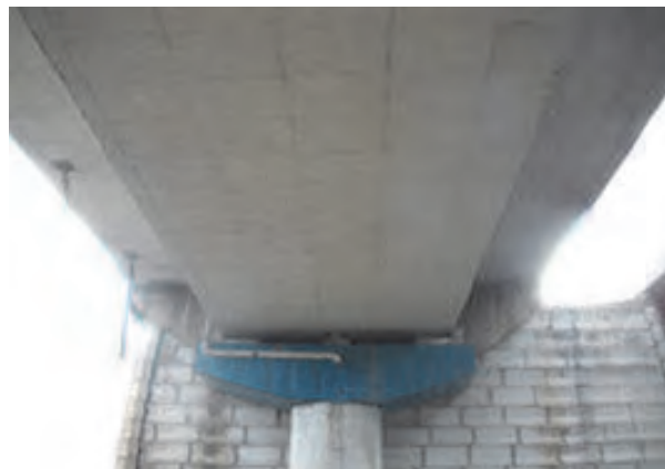
Photo 3.7.42 General View of LC No.2/A North
