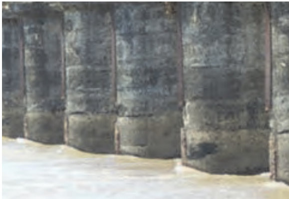
Photo 3.7.58 Repair of Damaged Pile
