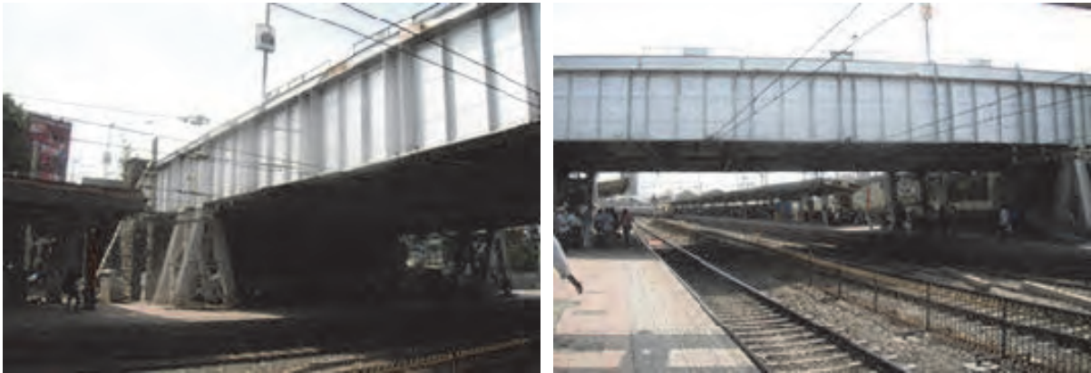
Photo 3.7.19 General View of Tilak ROB
