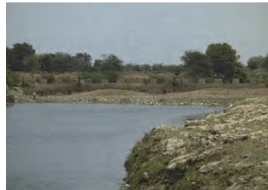
Photo 3.7.65 View of North side from Railway Bridges
