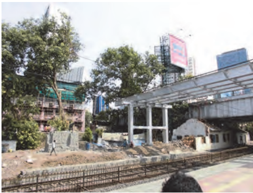
Photo 3.7.21 View of Southwest from ROB
