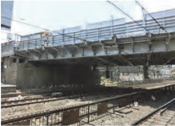
Photo 3.7.1 General View of Ferere ROB
