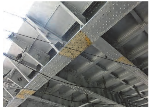
Photo 3.7.3 Main Girder and Cross Beam
