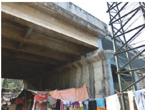
Photo 3.7.30 General View of Goregaon ROB
