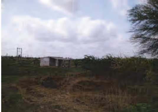
Photo 3.7.47 View of Southwest from North ROB
