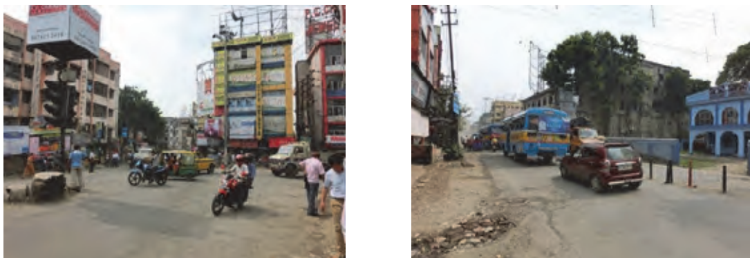
Photo 3.5.5 General View of Intersection between NH34 and NH35
