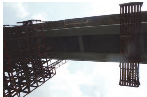
Photo 3.7.62 PSC I-Girder of No. 114 Bridge
