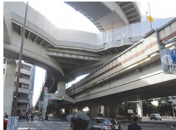
Photo 3.2.4 Nishi-shinjuku Junction (Tokyo-metropolitan)
