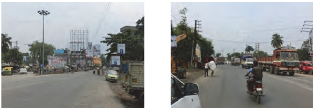
Photo 3.5.4 General View of Intersection between NH34 and Local Road
