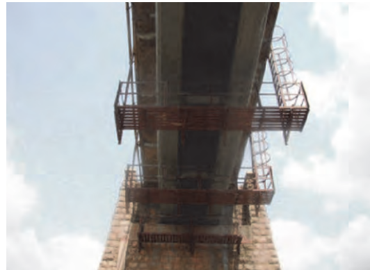
Photo 3.7.67 PSC I-Girder of No. 132 Bridge
