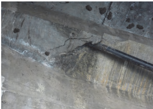
Photo 3.7.26 External Prestressed Cable
