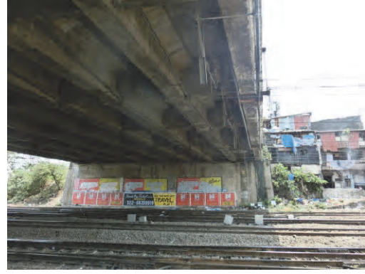
Photo 3.7.24 Main Girder and Abutment
