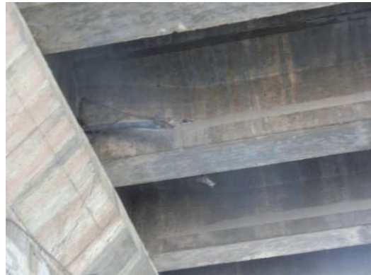
Photo 3.7.32 Cut external PC Cable
