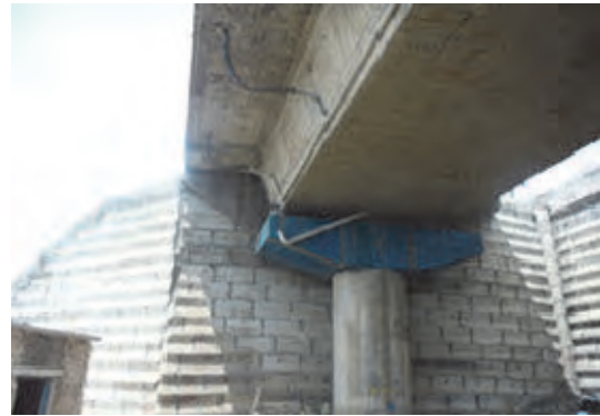
Photo 3.7.44 General View of LC No.2/A North
