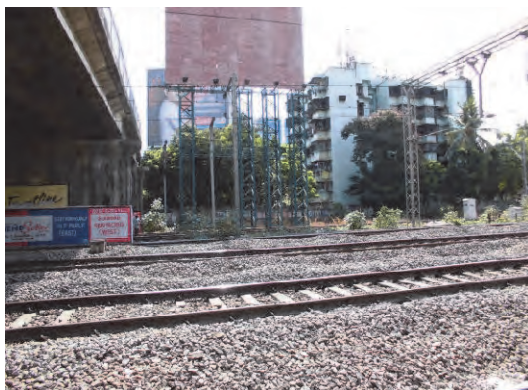
Photo 3.7.33 View of Northeast from ROB
