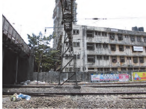
Photo 3.7.9 View of Northwest from ROB
