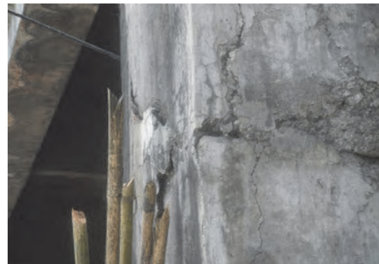
Photo 3.7.27 RC Pier Column
