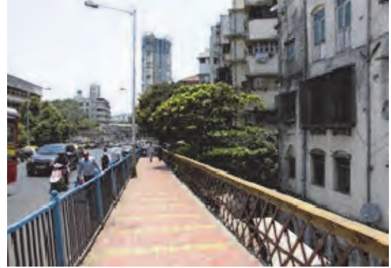
Photo 3.7.5 View of Northwest from ROB
