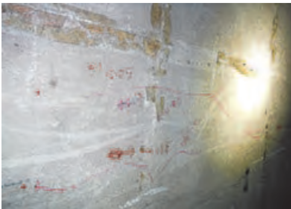
Photo 3.7.37 Cracks of Deck Slab
