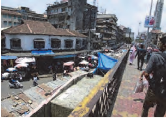
Photo 3.7.4 View of Southwest from ROB
