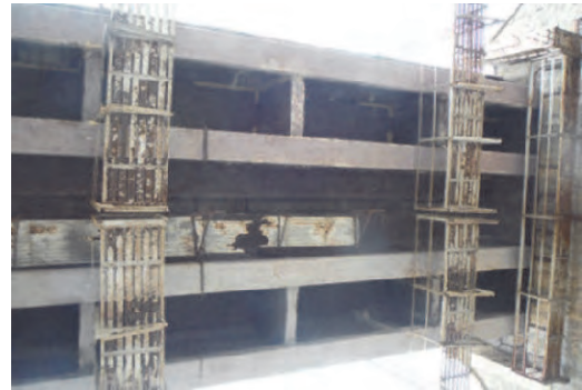
Photo 3.7.81 PSC I-Girder of No. R8 Bridge
