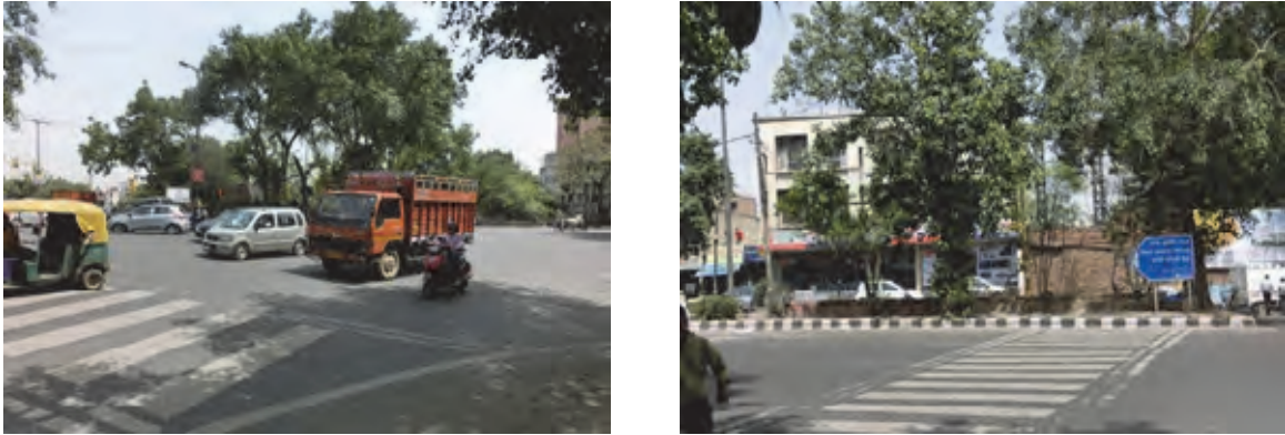
Photo 3.2.2 Existing Condition of Intersection between D. B. Gupta and Rani Jhansi
