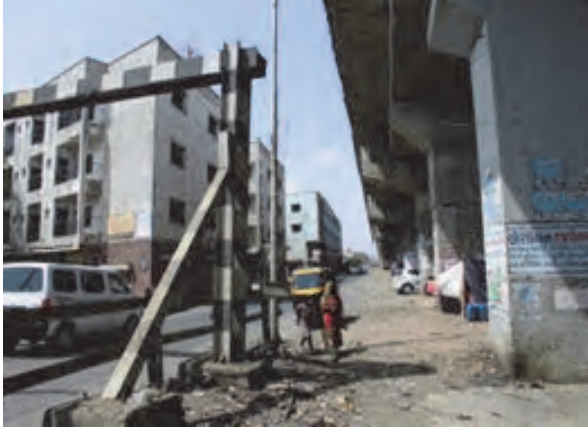
Photo 3.7.39 View of Northeast from ROB
