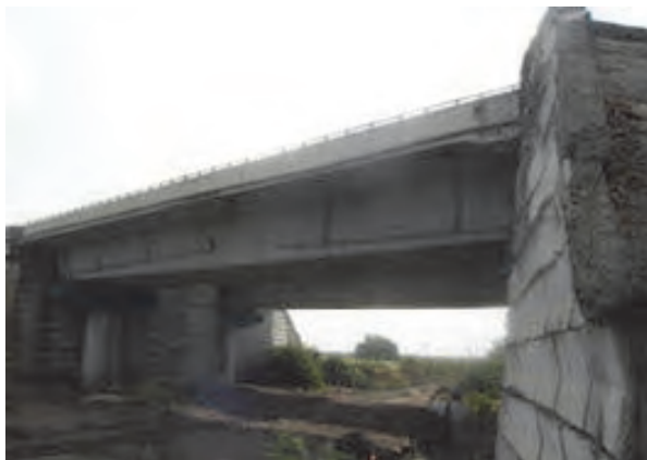
Photo 3.7.41 General View of LC No.2/A North
