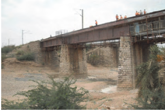
Photo 3.7.71 General View of No. 129 Bridge
