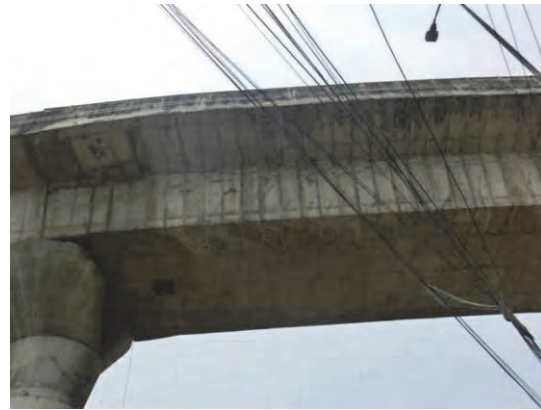
Photo 3.5.3 Horizontal and Inclined Cracks at Web
