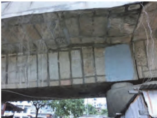
Photo 3.5.2 Mortar Filling
