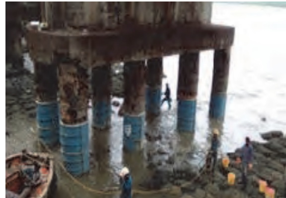
Photo 3.7.58 Repair of Damaged Pile
