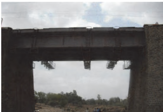
Photo 3.7.76 General View of No. R5 Bridge
