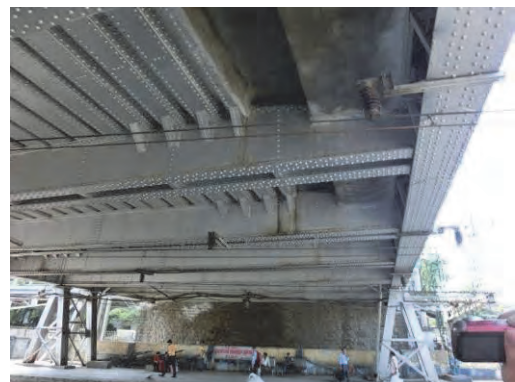
Photo 3.7.20 Main Girder and Cross Beam
