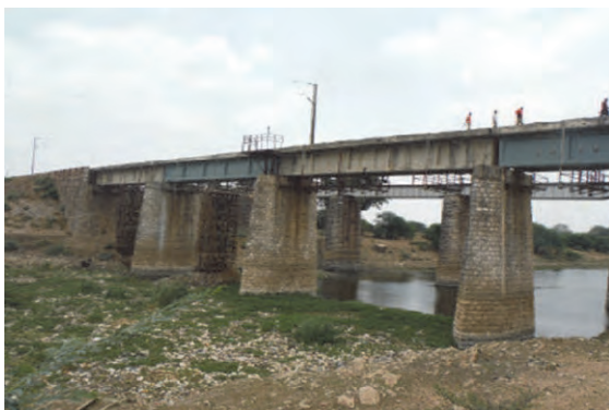
Photo 3.7.61 General View of No. 114 Bridge
