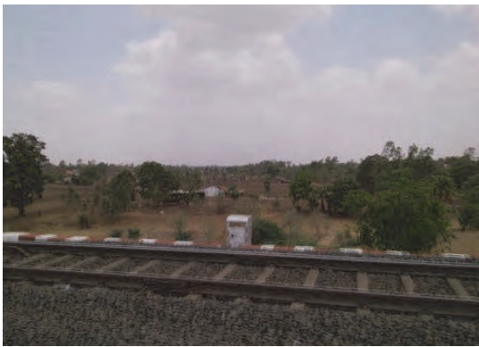
Photo 3.7.84 View of West side from Railway Bridges
