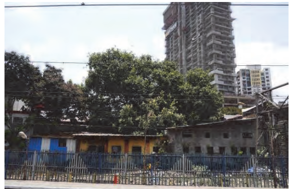
Photo 3.7.10 View of Southwest from ROB
