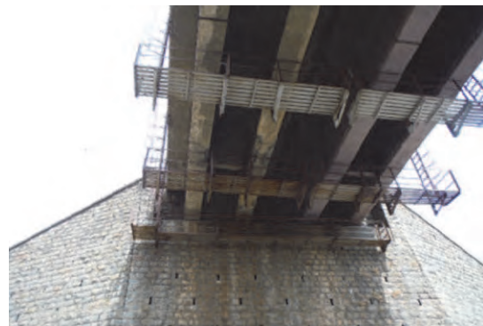
Photo 3.7.77 PSC I-Girder of No. R5 Bridge
