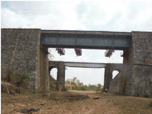
Photo 3.7.66 General View of No. 132 Bridge
