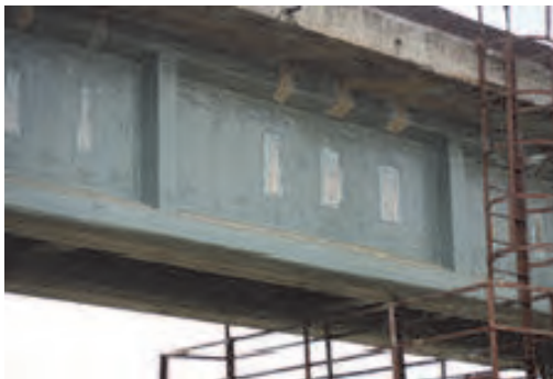
Photo 3.7.68 CFRP Epoxy Coating
