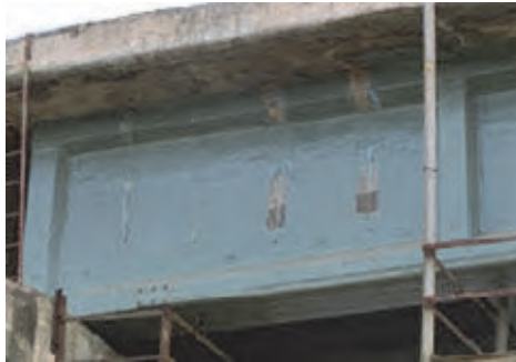
Photo 3.7.63 CFRP Epoxy Coating
