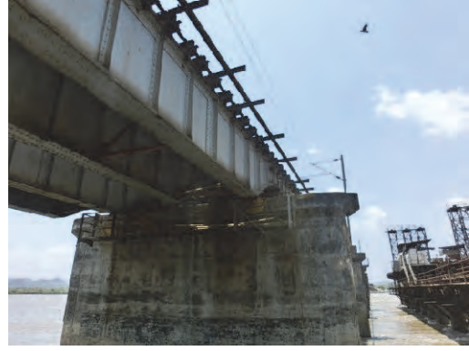
Photo 3.7.57 Girder and Pier Column
