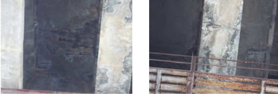
Photo 3.7.78 Exposed Reinforcement
