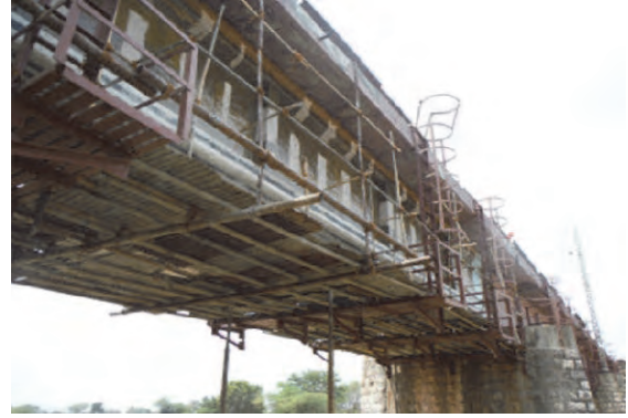
Photo 3.7.72 PSC I-Girder of No. 129 Bridge
