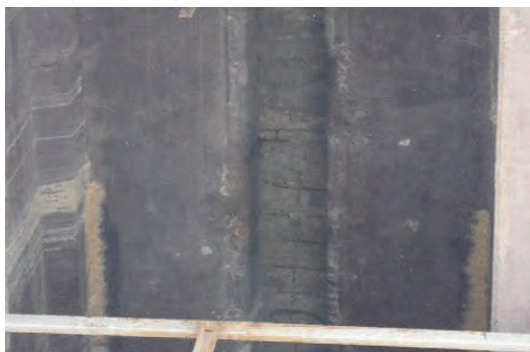
Photo 3.7.82 Exposed Reinforcement
