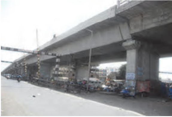
Photo 3.7.35 General View of LC No.5/A
