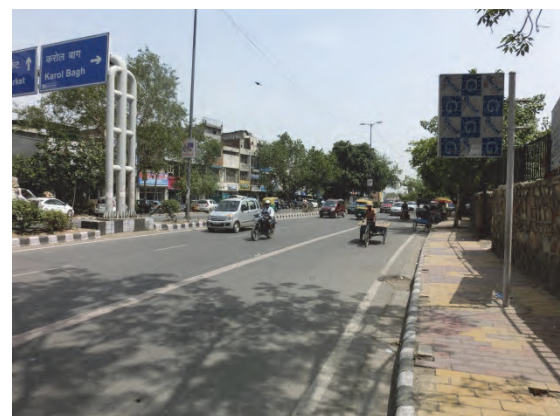
Photo 3.2.1 Current status of Rani Jhansi Road
