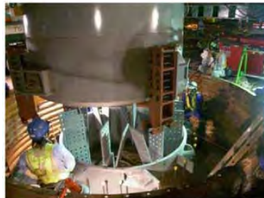
Connection part at tip of pier column
