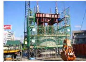
Construction of Caisson Structure
