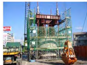
Construction of Caisson Structure
