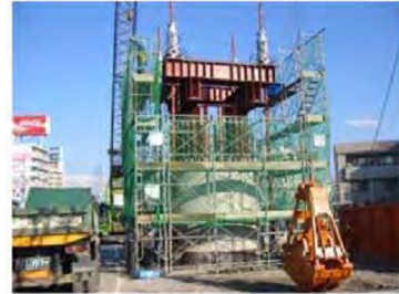
Construction of Caisson Structure
