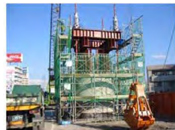
Construction of Caisson Structure
