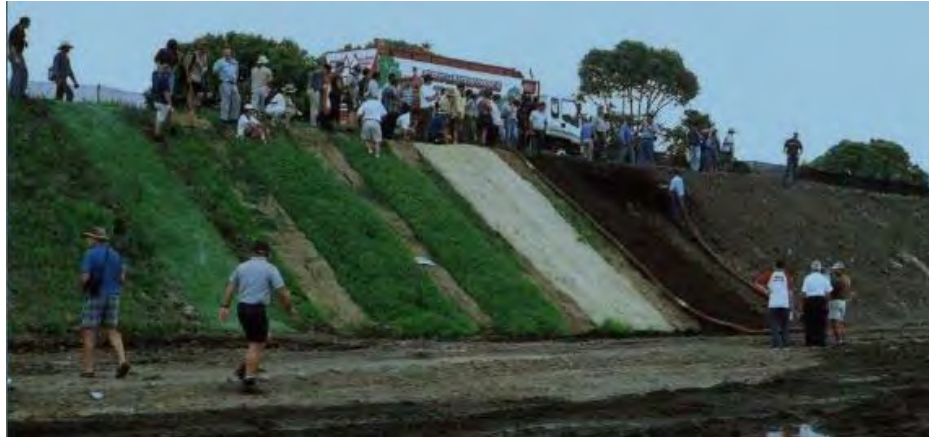
Photo : On site test for scattering clay soil measures
