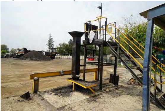
SA: Sampling from dump truck bed in Much Asphalt
