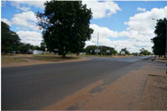
Zambia: Livingstone Road after repair (beginning point)
