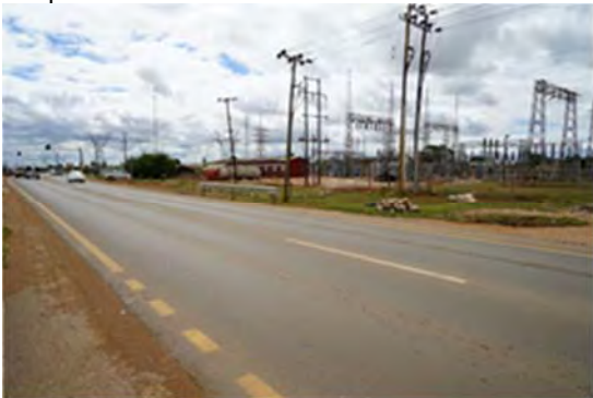
Zambia: Condition of “Tokyo way” in Lusaka (Fair)
