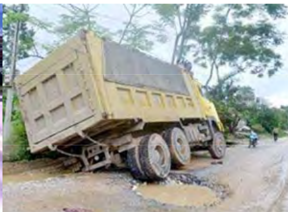
Pothole caused by overloaded vehicles
