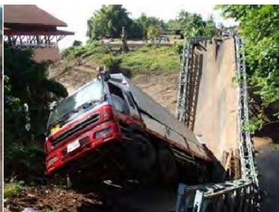
A bridge collapsed due to the overloading
