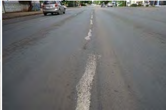
Zambia: Livingstone Road after repair (rutting at the intersection)
