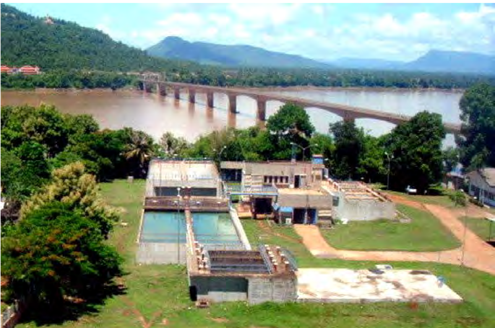
Champasack Province Km2 Water Treatment Plant (Photo)
