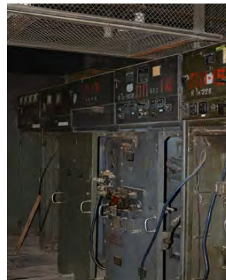
10kV indoor distribution switchgear
