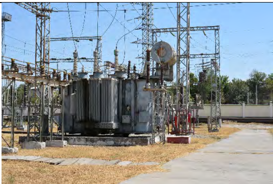
25MVA transformer
