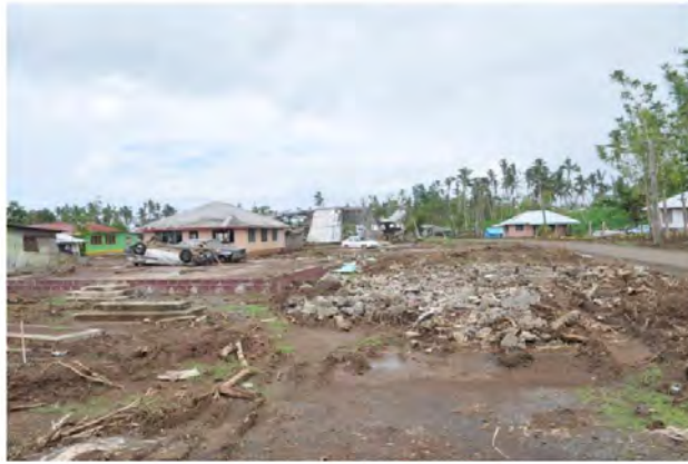
Figure 8 Damage to Houses and Cars at Lelata
