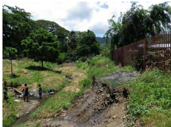
Embankment within the site
