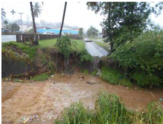
Drainage channel discharge mouth
