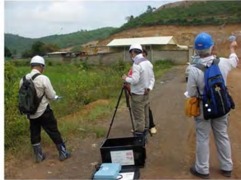
Measurement of vibration levels by blasting at the entrance of the quarry
