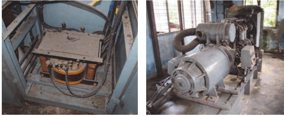
Figure 4.9.3 Step-up Transformer and Emergency Generator
