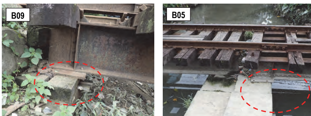
Figure 4.6.10 Unstable Bearing Structure
