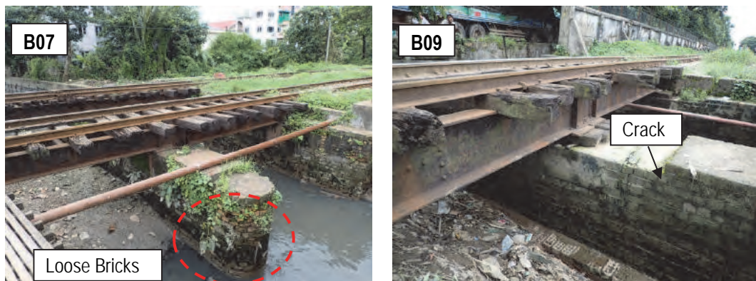
Figure 4.6.15 Substructure of Brick
