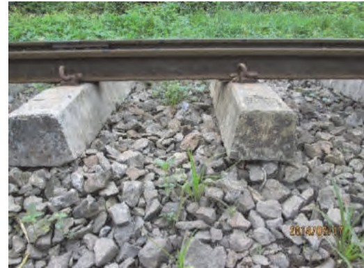
Figure 4.4.5 Ballast Condition
