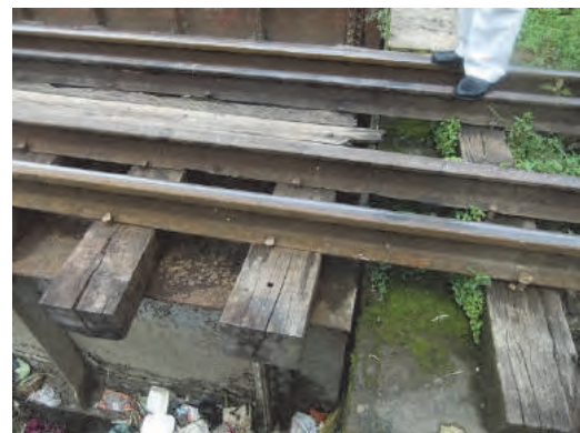
Figure 4.4.4 Wooden Sleeper at Railway Bridge
