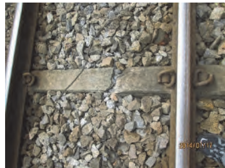
Figure 4.4.3 Damage on Sleeper made in India
