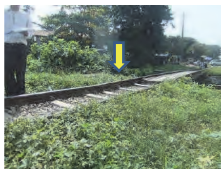
16km750m(W) Different Rai Level at rail Joint (27/Aug/2014)
