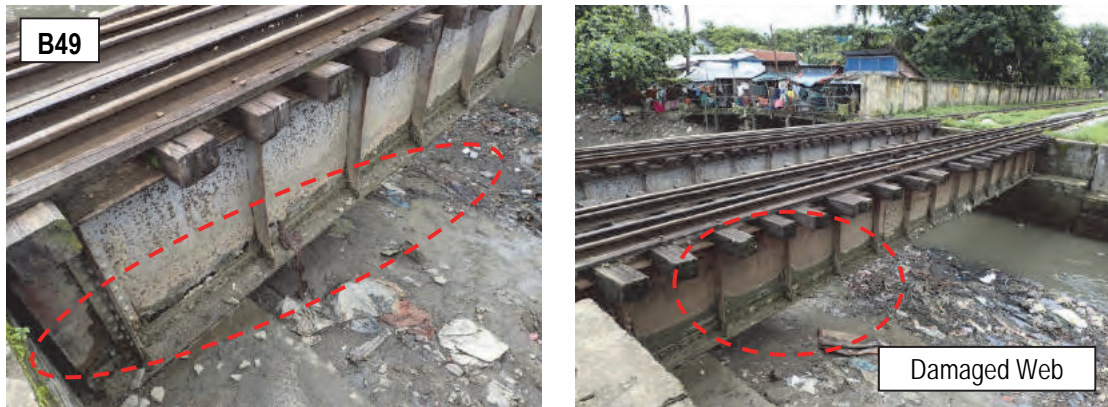
Figure 4.6.12 Traces of Water Inundation in B49
