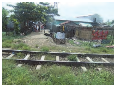
18km000m Nonsufficient ballast (27/Aug/2014)
