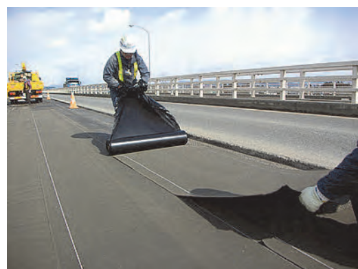
Figure 4.6.18 Construction of Water Proofing Sheet
