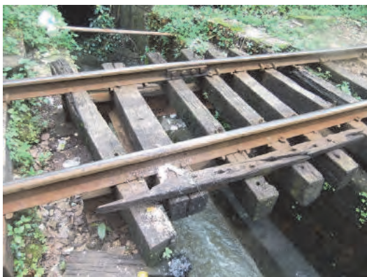
Figure 4.4.4 Wooden Sleeper at Railway Bridge
