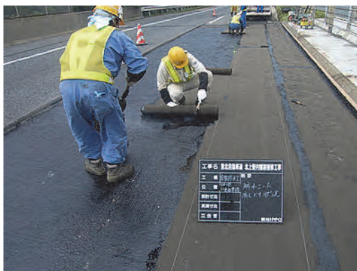
Figure 4.6.18 Construction of Water Proofing Sheet
