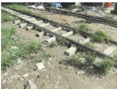
16km750m(W) Non Ballast and Mud Pumping (27/Aug/2014)
