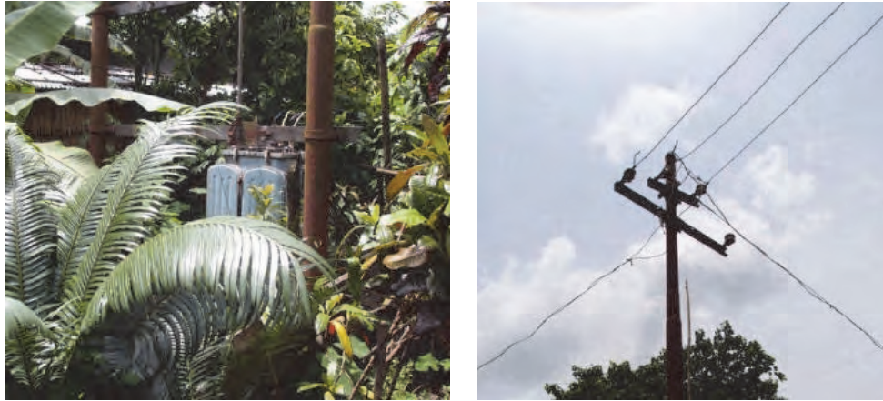
Figure 4.9.1 Old Transformer and Old Low Voltage Power Distribution Line
