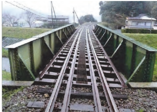
Figure 4.6.21 Picture of Steel Girder Bridge (Through Plate Girder)
