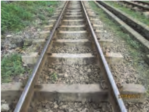
Figure 4.4.5 Ballast Condition
