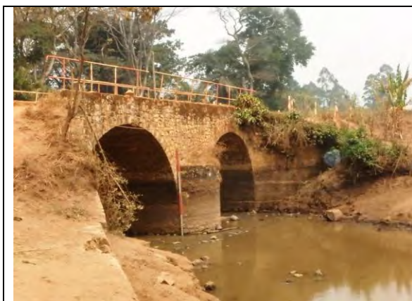
Arch-Shaped Stone Bridge
