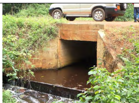
Box Culvert with Streambed Protection
