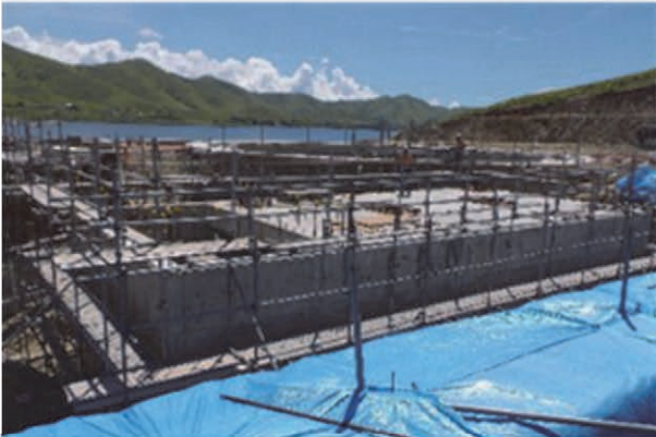
Sludge Pump Room #2- Roof slab casting complete
