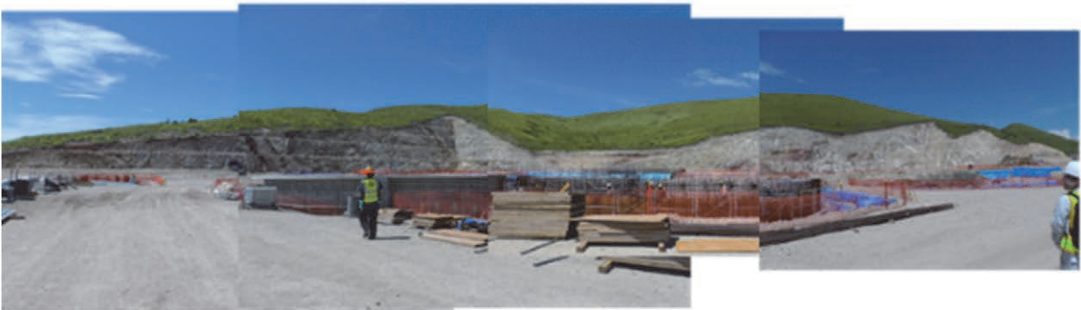
View of Slopes
