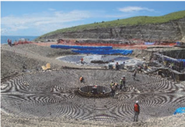
Final Sedimentation Tank- Re-bar works
