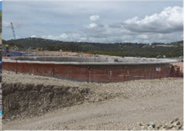
Final Sedimentation Tank #4- Wall casting complete
