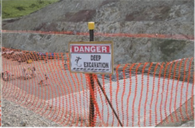
Safety Signage- Deep Excavation
