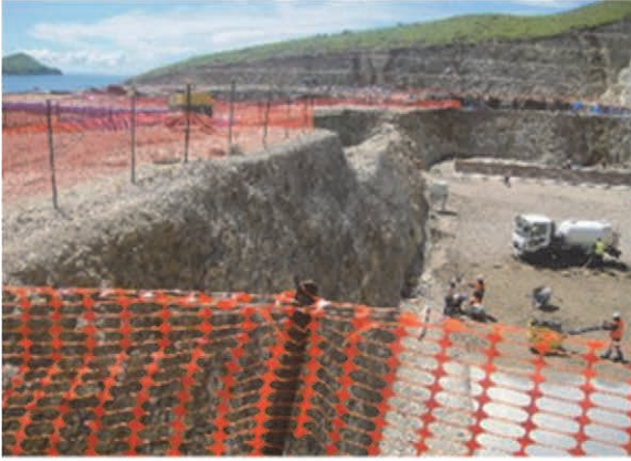
Oxidation Ditch- Foundation works
