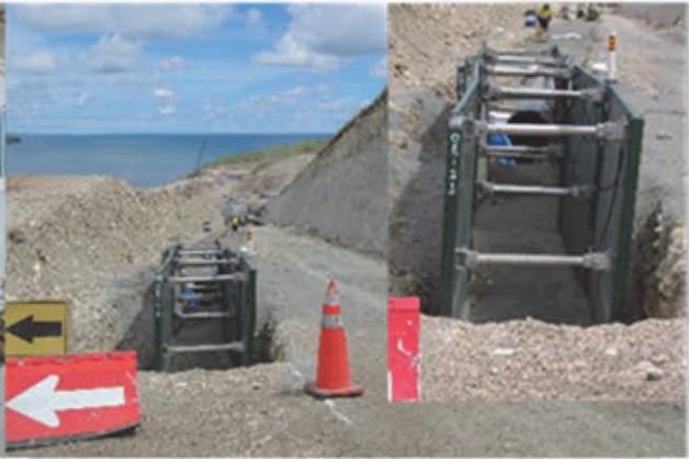
Retaining System for laying pipes
