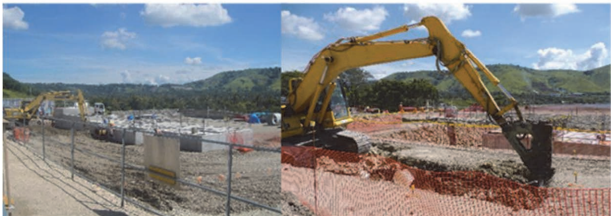
Grit Chamber- Backfilling
