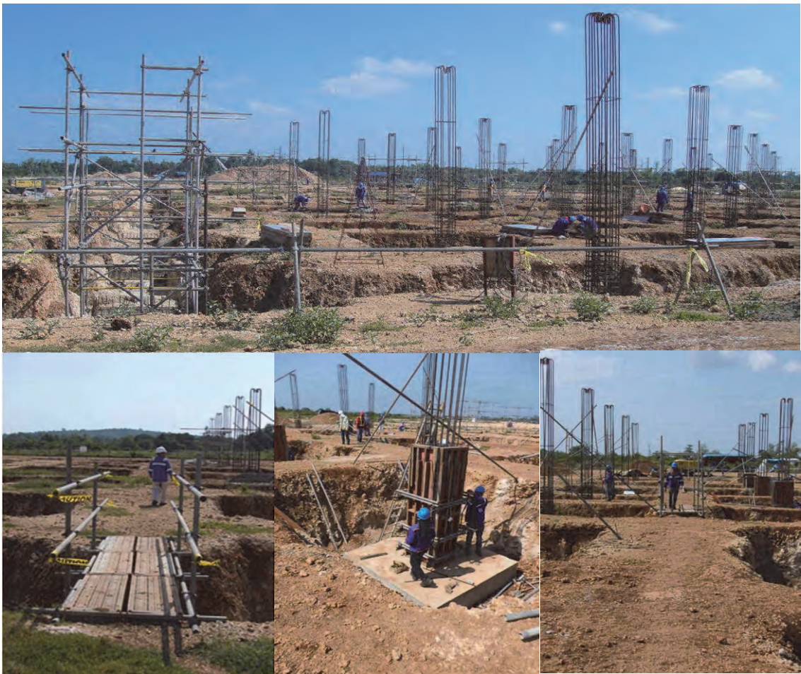
Figure 6-1 Excavation areas for independent footings of PTB
