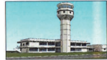
03 - Admin & CTO Building
