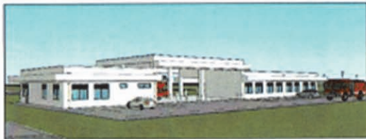
04 - Fire & Rescue and Maintenance Building
