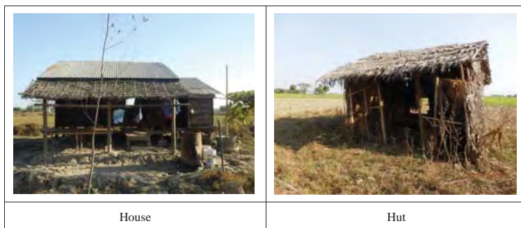
Photo 5-1 Example of House and Hut
