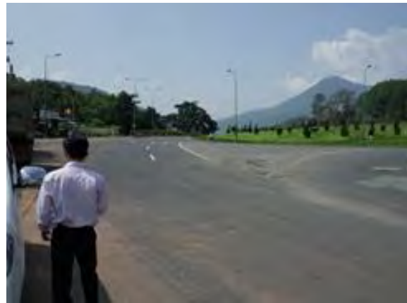
Figure 33: Connection point in front of Da Lat Flower Collection Center
