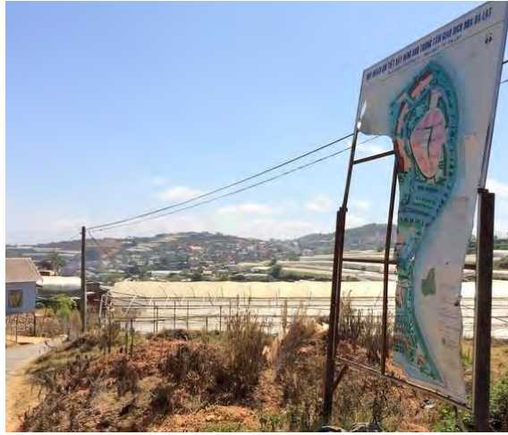
Figure 25: Signs indicate Da Lat Flower Wholesale Market construction site
