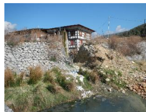
Pit of Embankment
