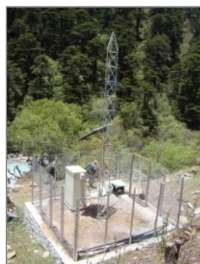
Water Level Station of Tsampa AWS
