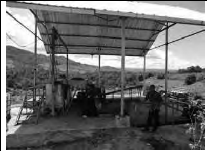
West Pakpak : Processing facility for Gambir
