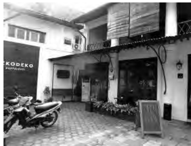
Photo 20: Kota Lama : Renovated historical building utilized for coffee shop
