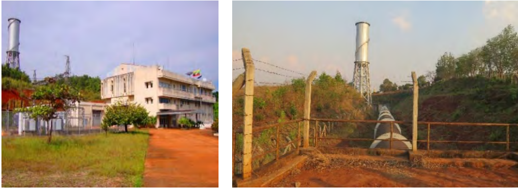
Photo 1 Existing Baluchaung No.1 HPP
