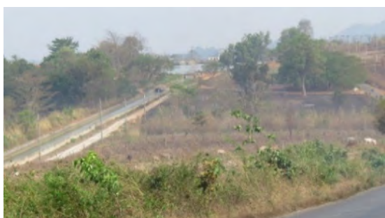
3) Waterway from Dawtacha Weir to the Pondage
