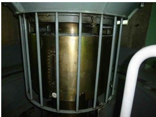
(1) Oil tank on turbine shaft
