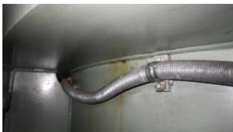
Oil Leakage from Welding Line
