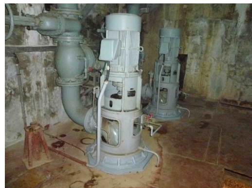
(2) Drainage pumps for draft tube dewatering pit
