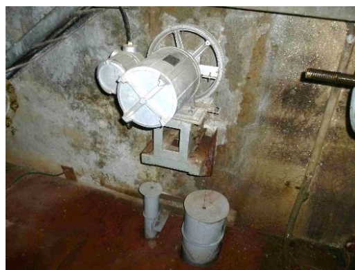
(2) Water level detector for drainage pit
