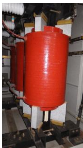
Photo 5.1-10 Excitation Transformer
