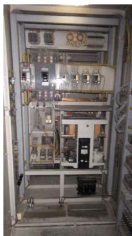
Control Panel of Exciter
