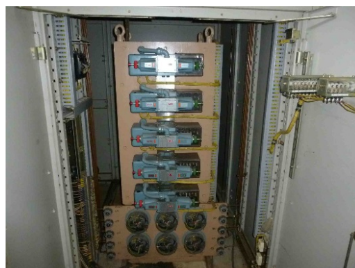
(2) Solenoid valves in turbine control panel
