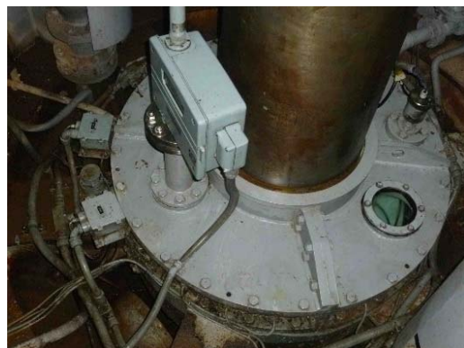
(2) Oil level detector and devices
