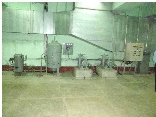
(1) Compressed air equipment
