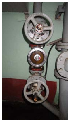
Flow Meter of Oil and Water (Value is Unread)
