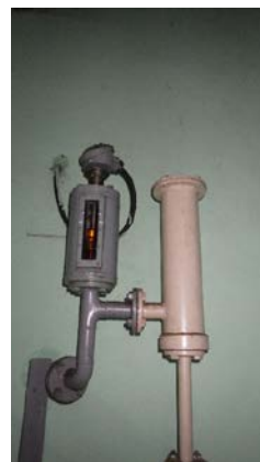
Oil Gauge of the Lower and Upper Thrust
