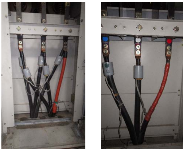
Photo 5.1-23 Repair of 11kV Power Cable
