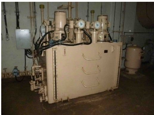
(1) Oil sump tank and related components
