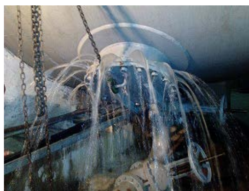
(2) Water leakage of unit #1
