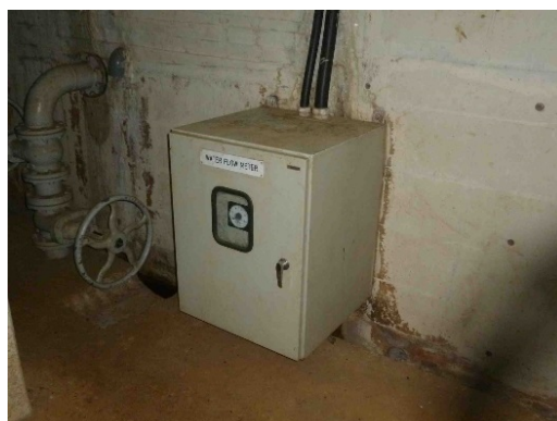
(2) Turbine flow meter transducer
