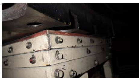
Unit-1 Splash protection materials of brake powder are partially in touch with the brake ring
