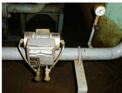
(2) Flowmeter at cooling water pipe
