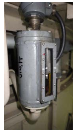
Oil Gauge of the Lower and Upper Thrust
