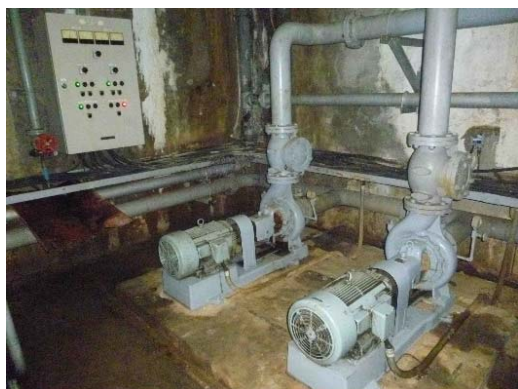
(1) Cooling water pumps
