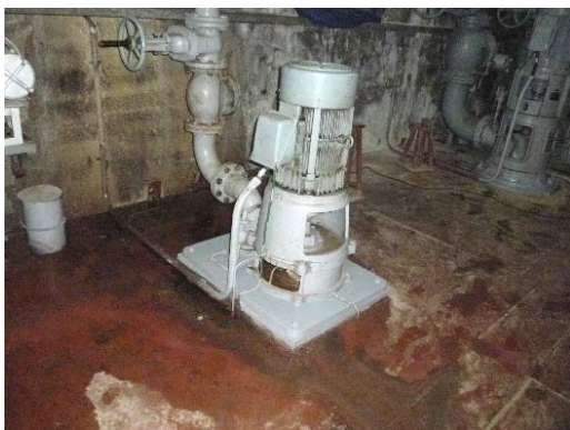
(1) Drainage pumps for powerhouse water leakage pit
