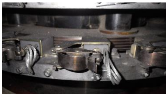
Carbone Brush Powder Slight Roughness at Lower Slip Ring Oil Leakage from Upper Bearing
