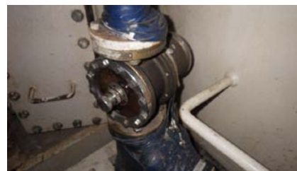
Flow Meter of Cooling Water (Electric Wire is unconnected)
