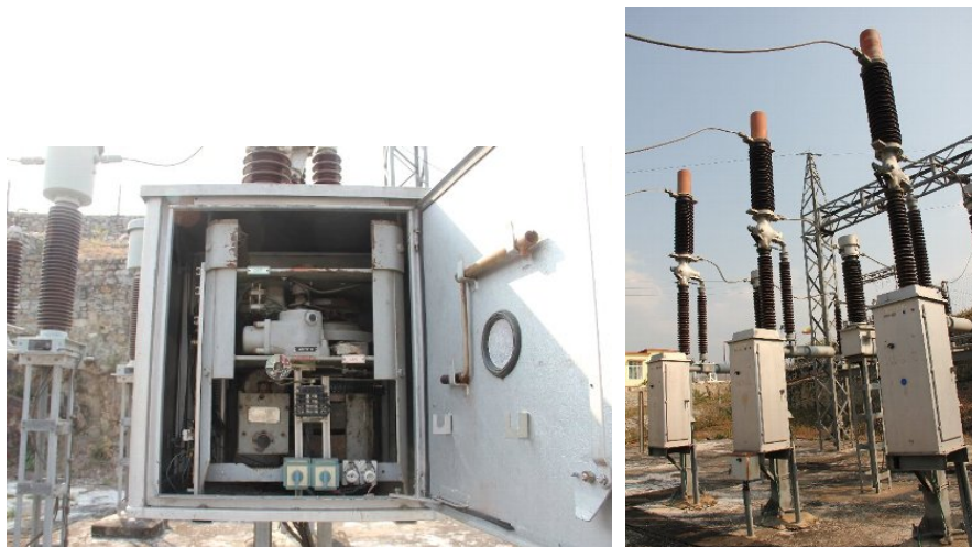
Photo 7.1-9 132 kV Switchgear
