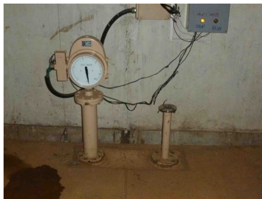
(2) Water level gauge/detector for the drainage pit
