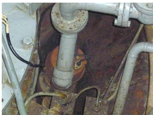
(1) Drainage pump on head cover (2 pumps/unit)
