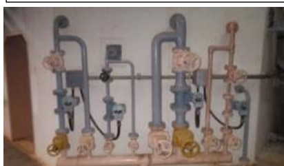
Discharge Meter of Cooling Water
