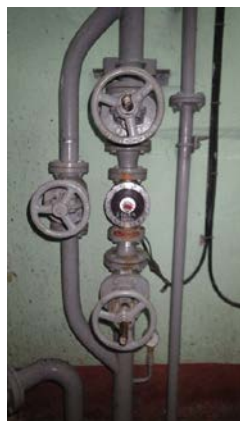
Flow Meter of Oil and Water (Value is Unread)
