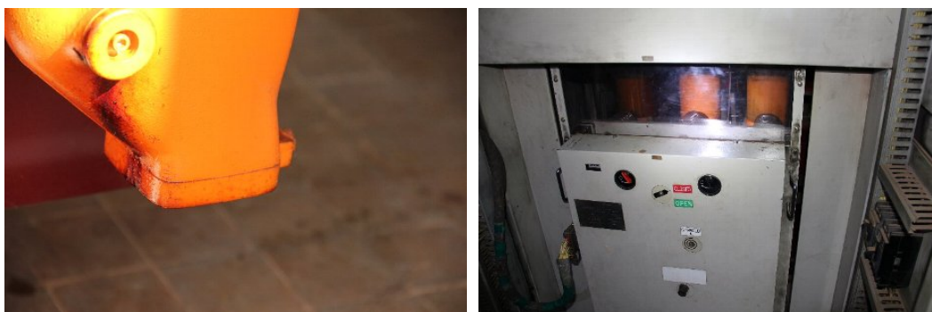
Photo 7.1-4 11 kV Switchgear (LOCCB)
