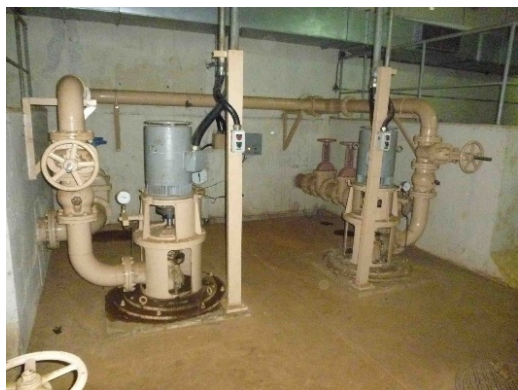
(1) Water drainage pumps for the drainage pit (regular use and backup)
