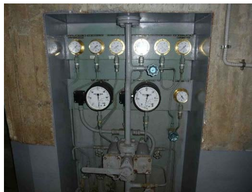
(2) Water pressure gauges/relays
