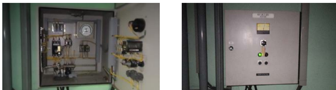
Photo 5.1-19 Generator Heater
