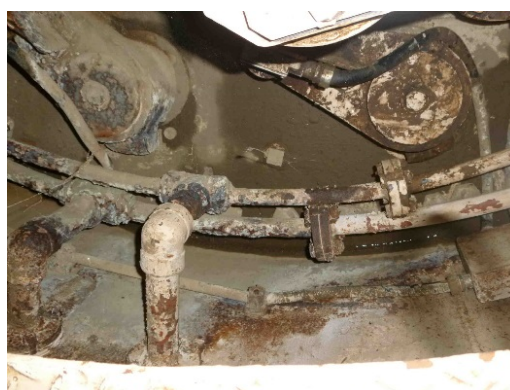
(2) Eroded water piping
