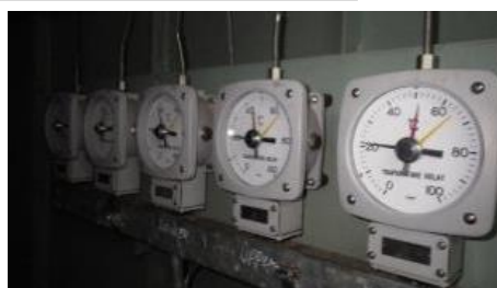
Dial Thermometer for each Bearing
