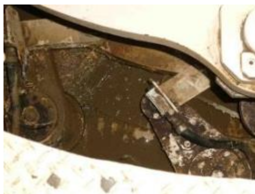
(1) Guide vane operating mechanism
