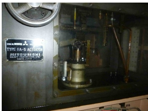
(1) Governor actuator portion in governor control panel
