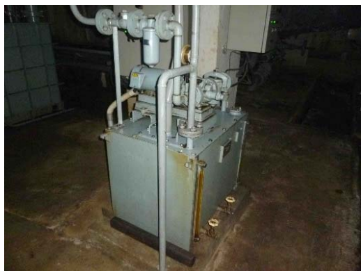
(1) Leakage oil tank set
