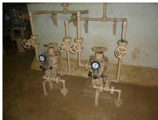
(2) Hand-operated water strainers (Regular use and backup)
