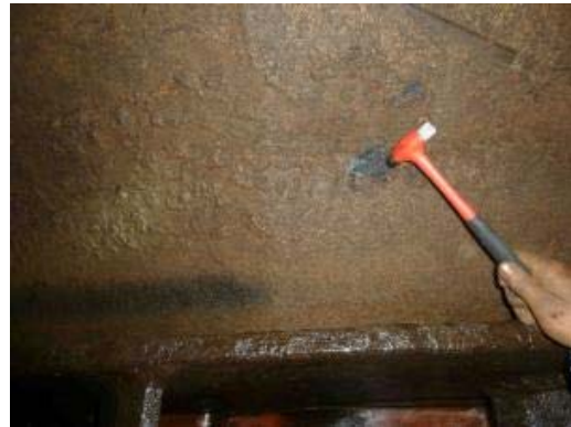
(2) Hammering check of rusty portion
