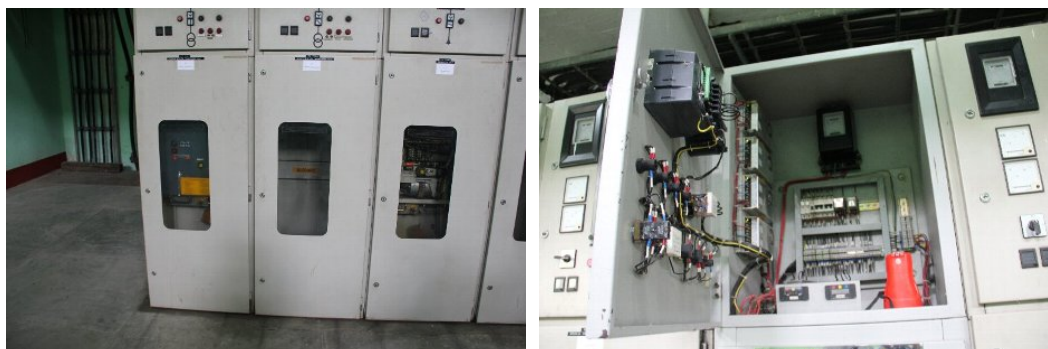
Photo 7.1-10 11 kV Switchgear
