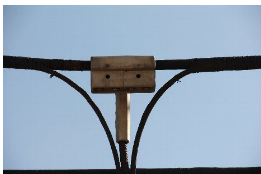
Photo 7.1-3 11 kV Busbar and Cable Clamp
