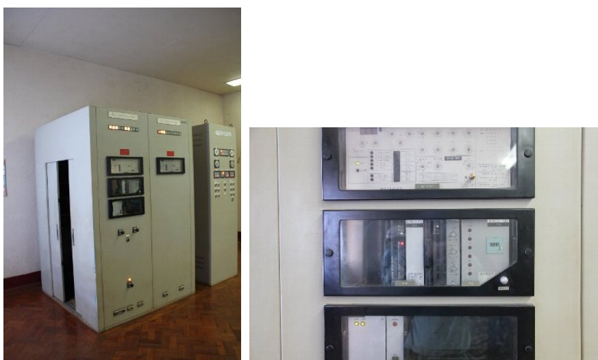
Photo 7.1-7 Transmission Line Protection Panel
