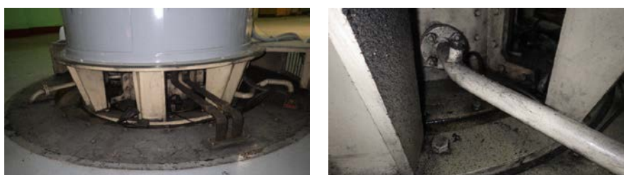
Oil Leakage at Upper Bracket
