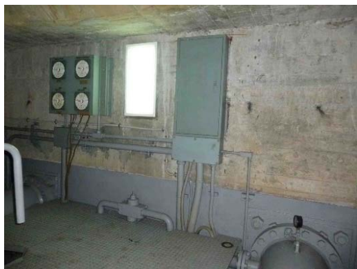
(1) Temperature indicators/relays
