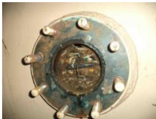
(2) Foreign Materials at the intake of cooling water piping
