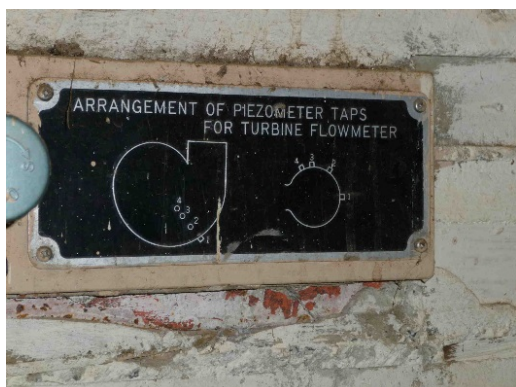
(1) Name plate for piezometer taps
