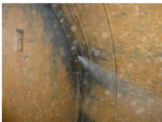
(1) Splashing water leakage (unit #1)
