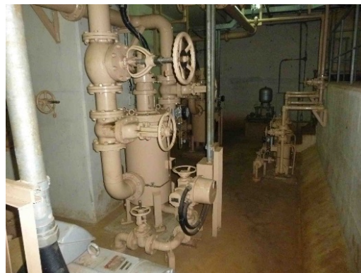
(1) Automatic water strainers (Regular use and backup)
