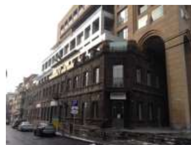
Photo: Renovation of historical building (Yerevan)
