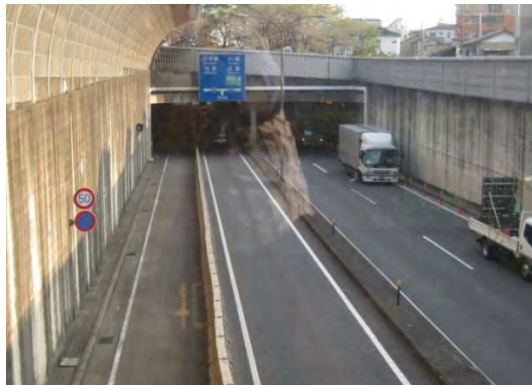
Photo 2.2.2-1 Example of Depressed and Underpass Section
