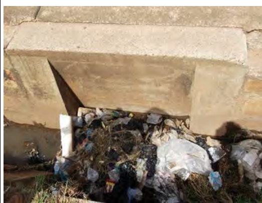
Clogging of drainage facilities
