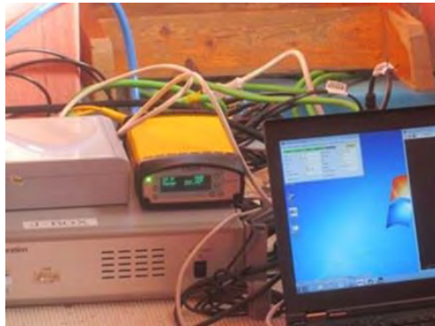
Upper left: Sonar controller modem, Center: GNSS receiver, Lower left: Power and signal convergence system
