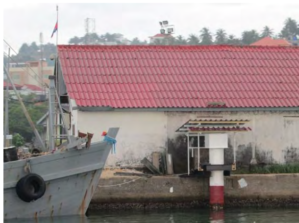
The distance view of Tide Station.
